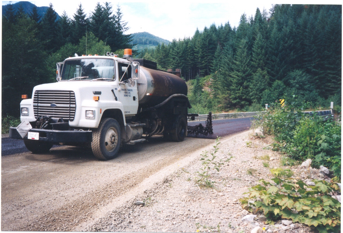
Spraying the Cationic Prime
