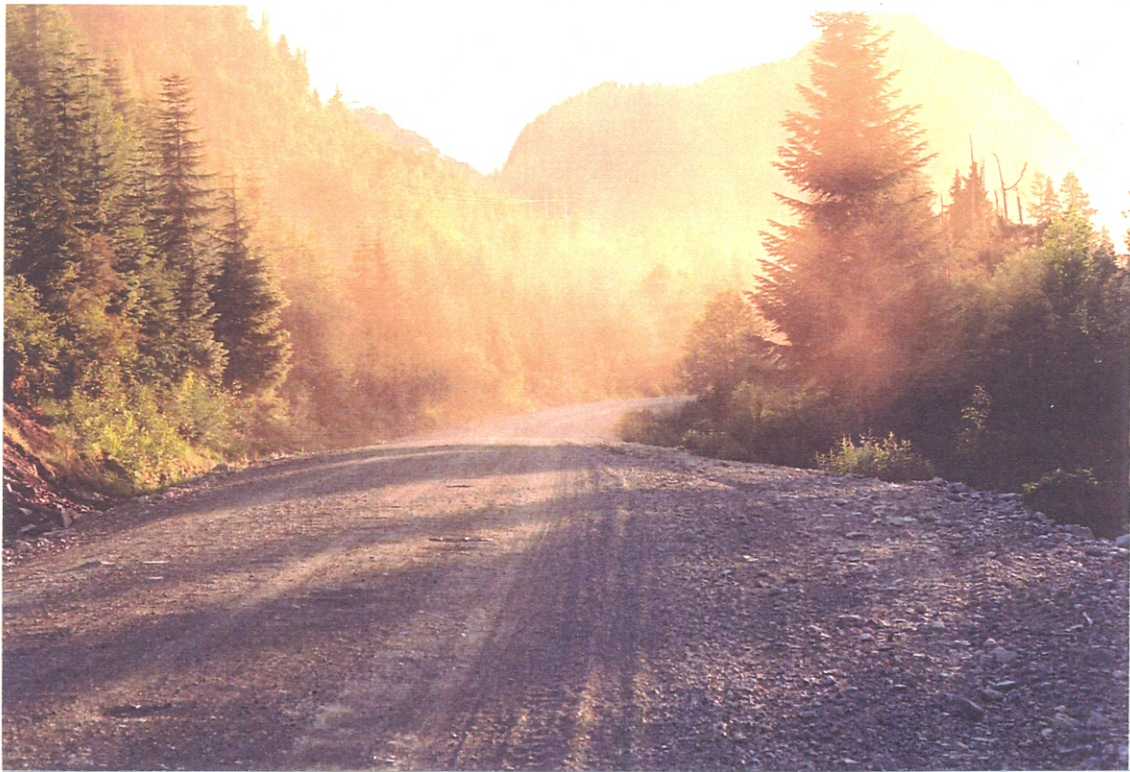
Typical section of the Tahsis Road – Dust, potholes, washboard and loose gravel
