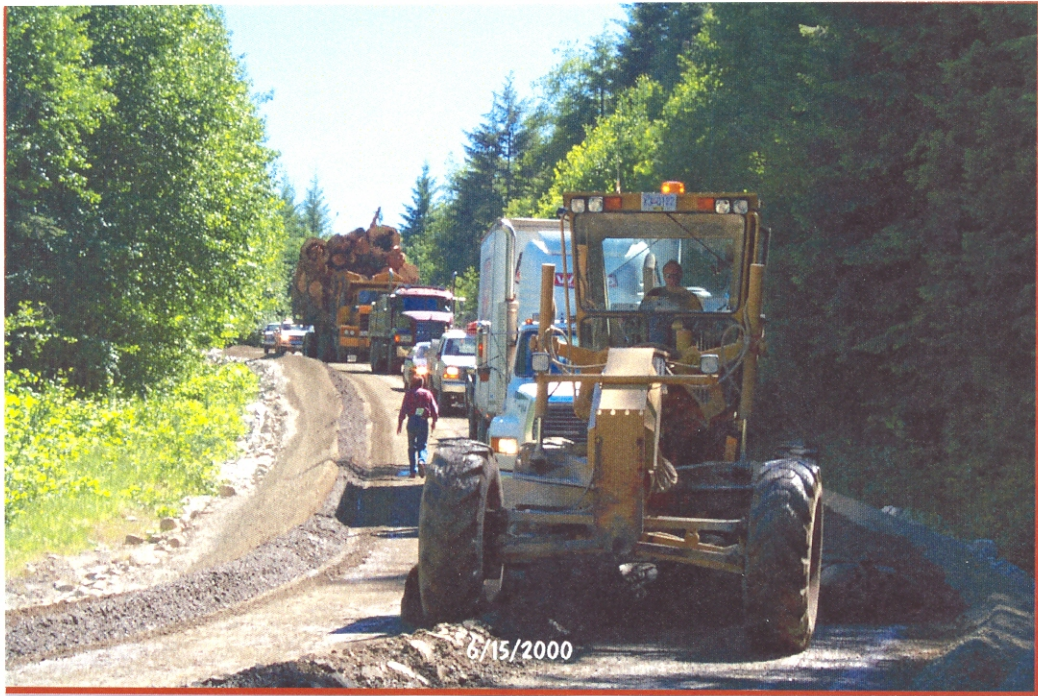
Grading in the MgCl - Freight truck, gravel truck and loaded logging truck on return trip
