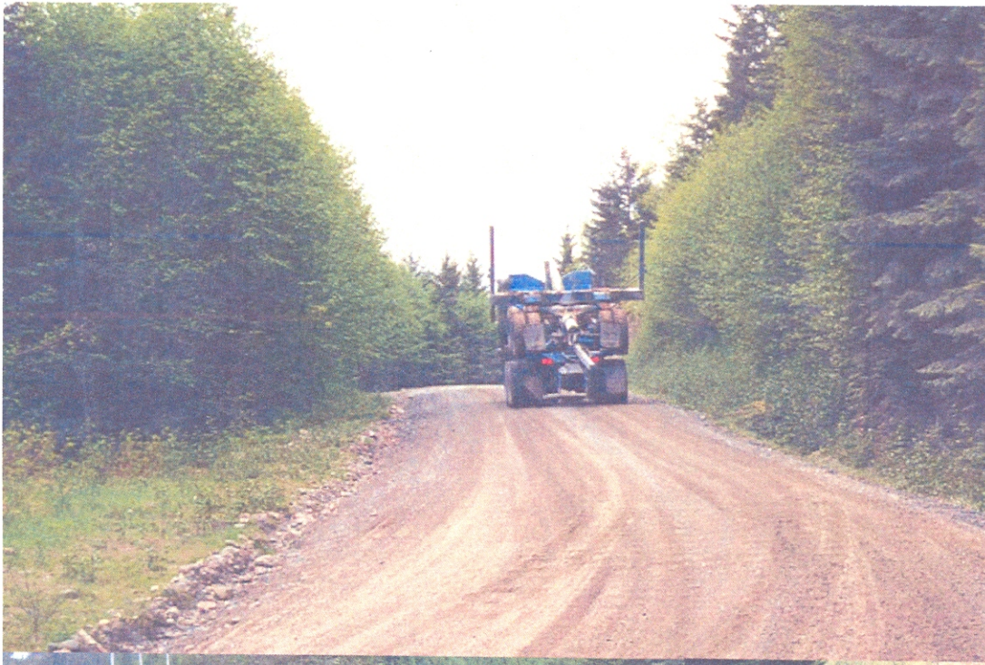
A section of the Tahsis Road treated with MgCl - One of Western's logging trucks headed for a load
