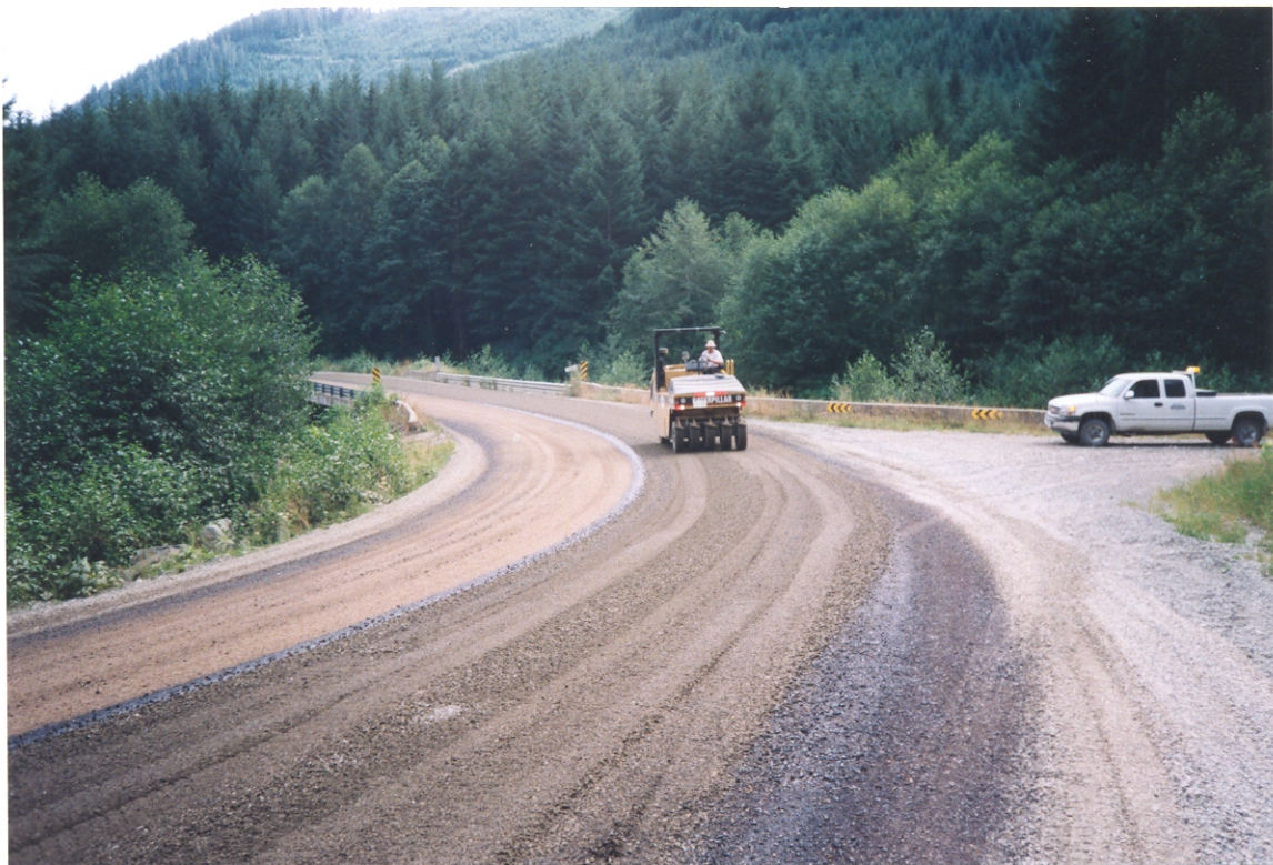
Rolling the first lift of Graded Aggregate Seal. On the left, the sand over the CSS 1 sealed section is quiet dry and being rolled smooth by the traveling public.
