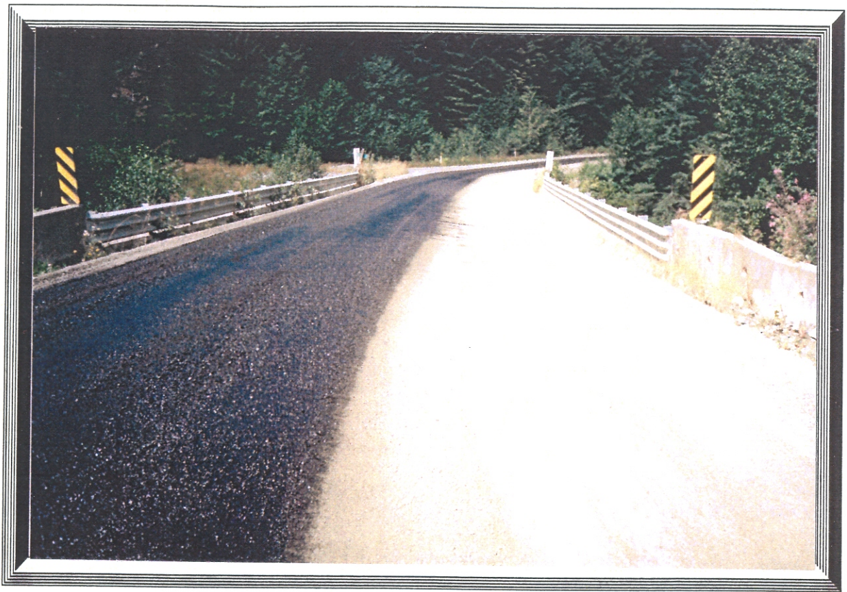
CSS1 (on the left) applied over MgCl stabilization. Application was a mixture of 0.5 litres CSS1 and 0.6 litres water per square metre.
