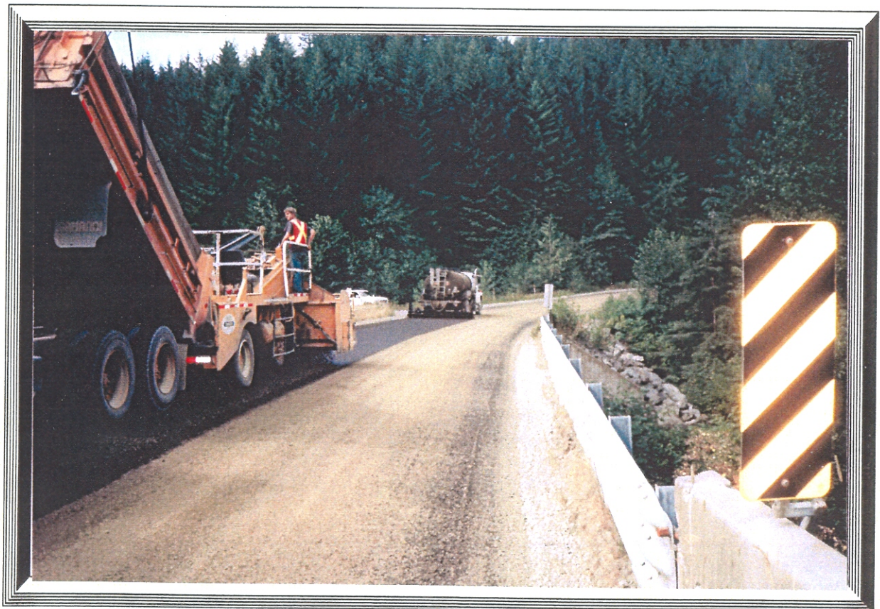
On the right a sand cover applied over the CSS1 that permits single lane traffic to be maintained. On the left, Shades Tanker Services applies bottom lift Class A Graded Aggregate Seal.
