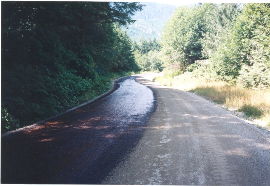
The dreaded early morning shaded section. After 20 minutes the product is still liquid and not cured.
