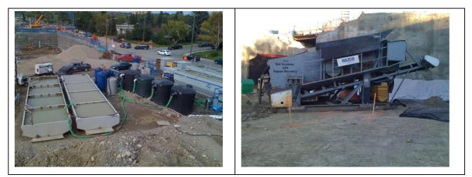
Photo 6 (L) Groundwater treatment process; Photo 7 (R) Soil screening process at Westbrook
