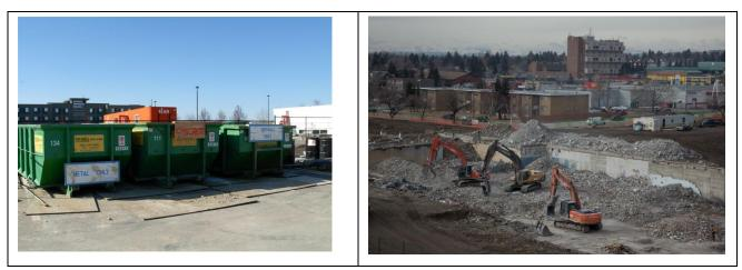
Photo 8 (L) Construction material waste stream separation; Photo 9 (R) Demolition waste stream separation
