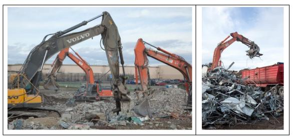
Photos 10 & 11: Demolition contractor separates reinforcing steel from concrete for recycling of both
