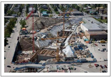
Photo 5: Excavation at Westbrook for the LRT line and station underground
