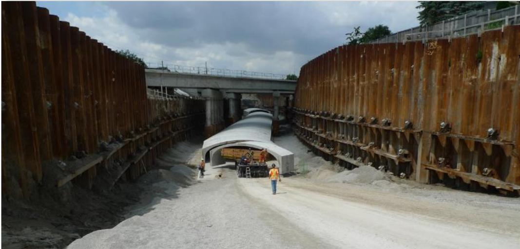
Photo #6 – Completed sheetpiling, subsequent excavation and storm retention tank
