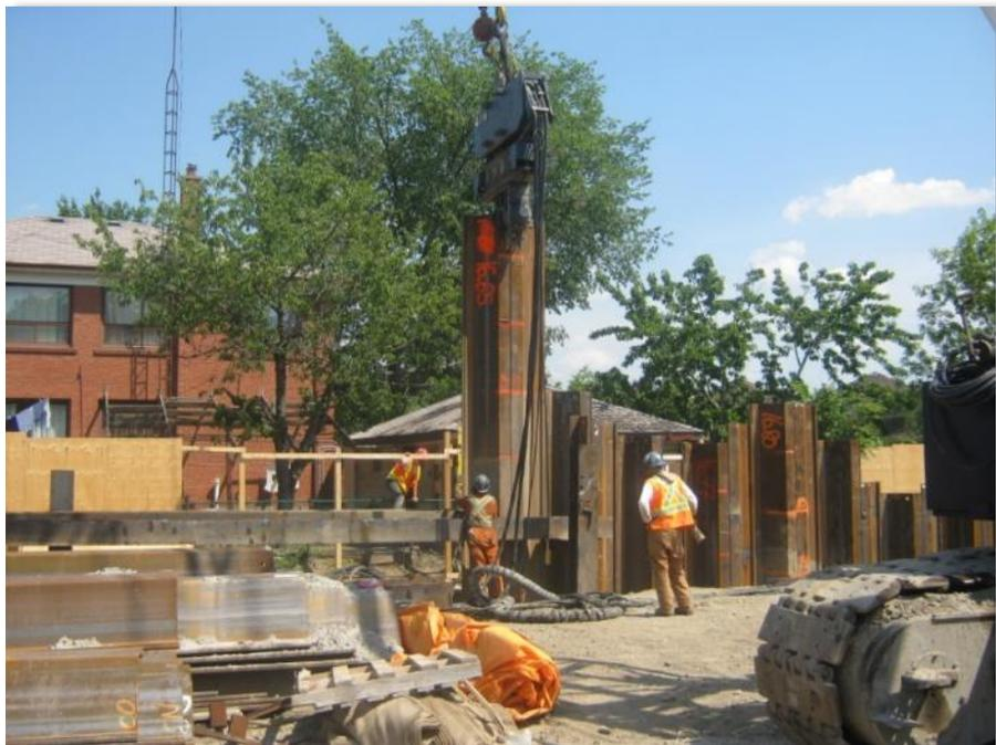
Photo #3 – Installing sheetpiles after pre-augering
