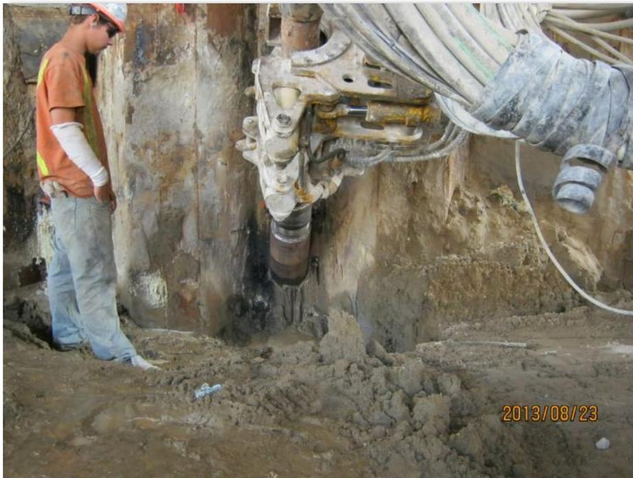
Photo #5 – Triple grout method
