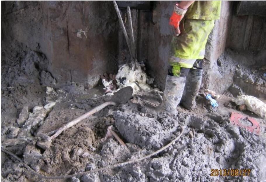
Photo # 4 – Foam application to prevent loss of fines
