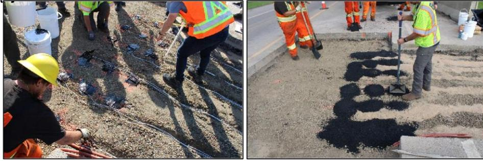
**Figure 12. (a) laying of vertical and horizontal asphalt strain transducers and (b) using hot mix asphalt to secure the transducers in place before resurfacing**
