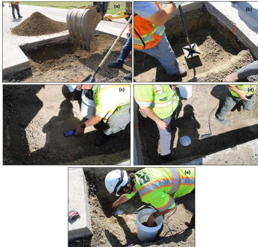
**Figure 10. Installation of the EPCs: (a) Removing the existing base layer (b) sand filling and compacting with a tamper, (c) checking for levelness of compacted sand, (d) laying the pressure cells and (e) covering pressure cells with sand**
