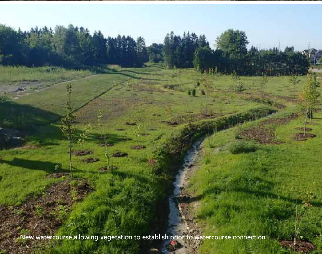
Upper reach constructed using bioengineering techniques to mimic headwater streams
