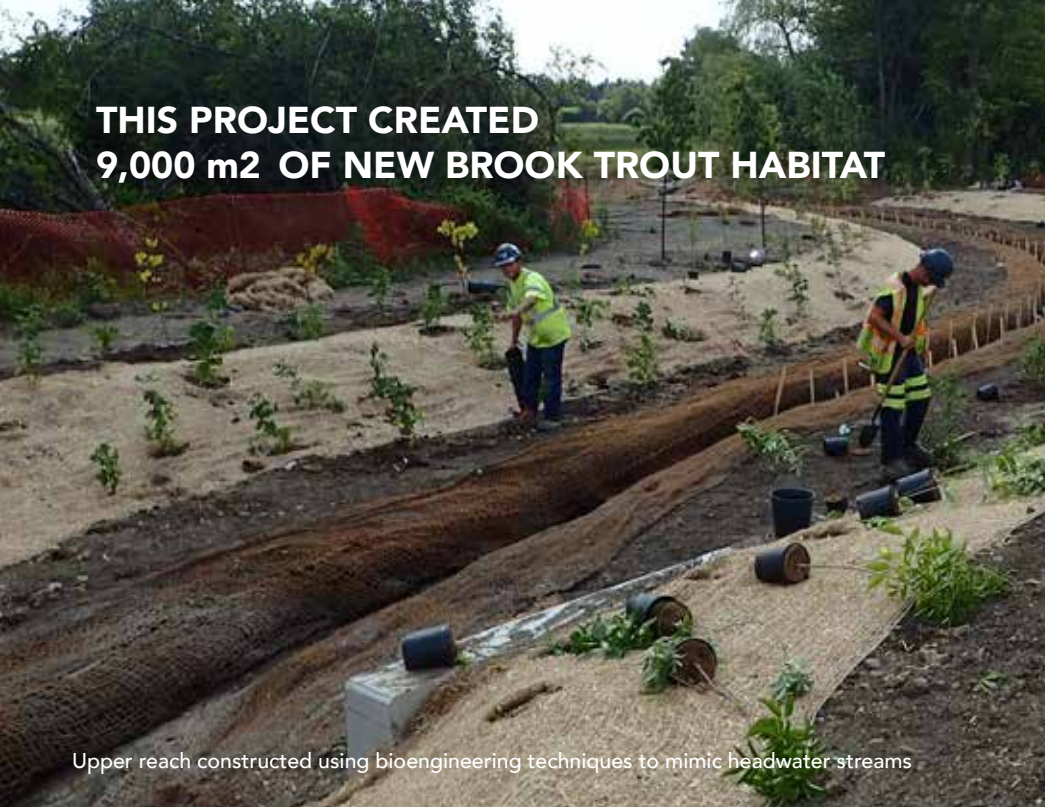
Live fascines in constructed watercourse
