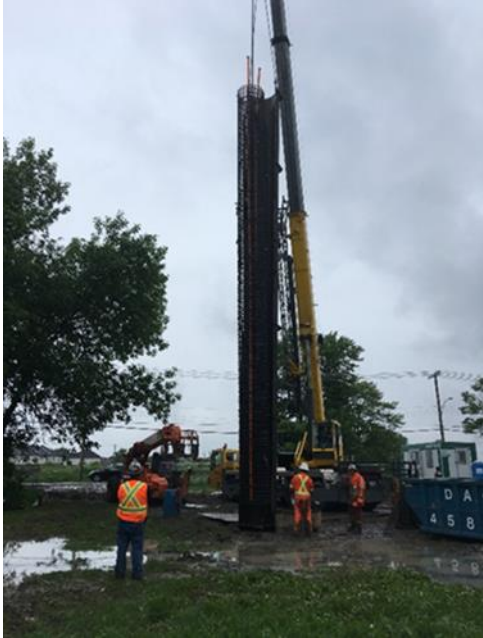
Figure 2: casing and cage placement
