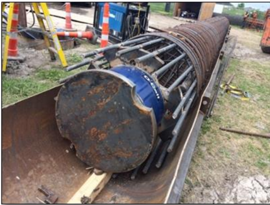
Figure 4: Rebar cage with attached O-cell
