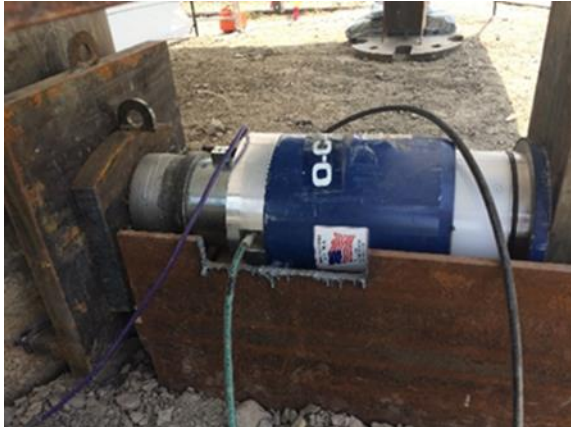
Figure 3b: O-cell for lateral load test
