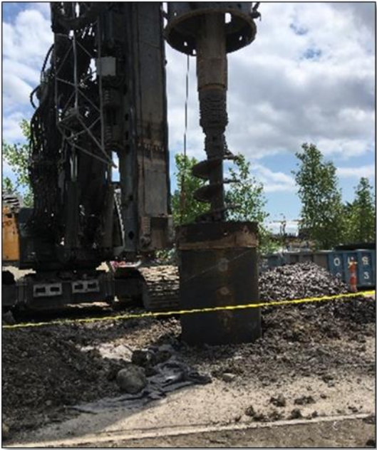
Figure 2: casing and cage placement
