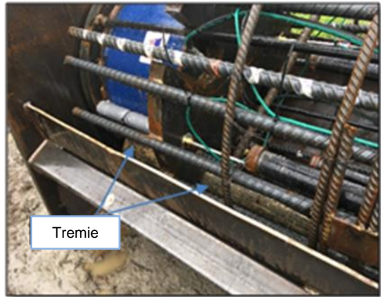
Figure 4: Rebar cage with attached O-cell
