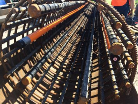
Figure 3a: Rebar cage with inclinometers
