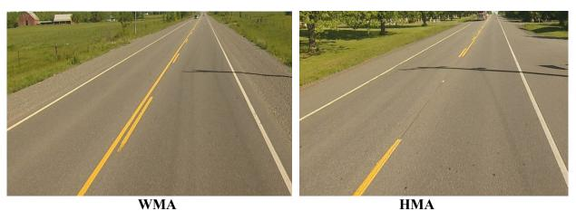
Figure 15 – Typical pavement condition on Highway 15 (paved in 2008)
