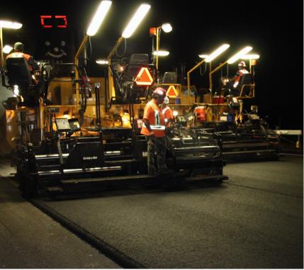
Figure 4 -Warm mix asphalt night paving - No visual emissions
