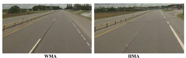
Figure 16 – Typical pavement condition on Highway 11 (paved in 2010)
