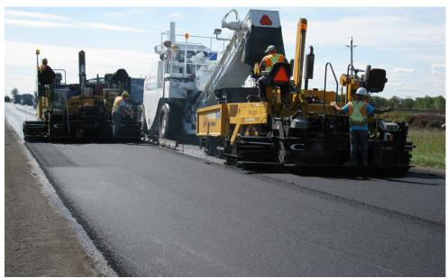
Figure 3 -Warm mix asphalt paving site - No visual emissions
