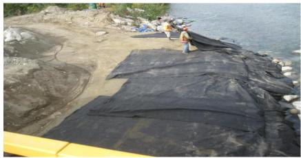
Figure 9: Building foundation and placing of geotextile
