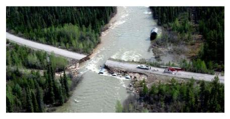
Figure 1: The Nahanni Range Road, which leads to the mine, was washed out in three locations. (Yukon Department of Highways and Public Works)
