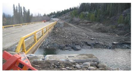
Figure 13: Bridge after placing on lock blocks
