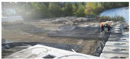
Figure 11: Placing of Geogrid
