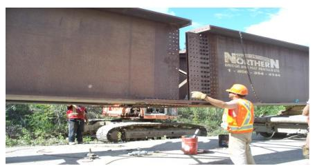
Figure 4: Two sets of girders to be spliced together on top of two trucks
