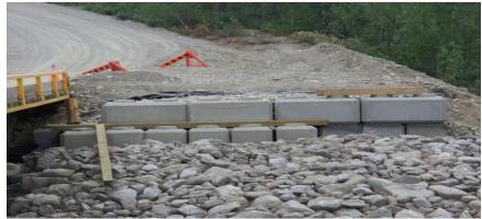
Figure 12: Half of permanent abutment
