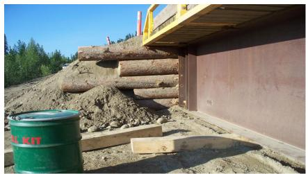
Figure 7: Temporary back wall made of trees
