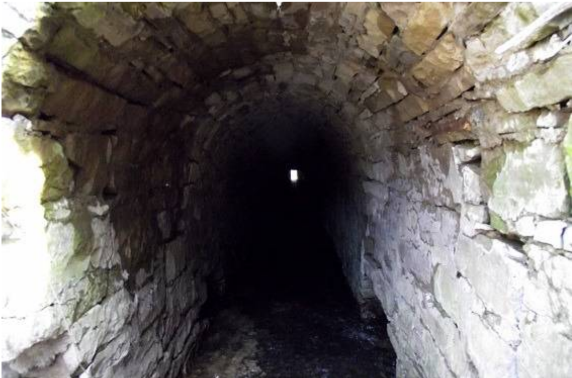
Figure 6 - Culvert Barrel
