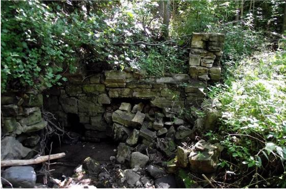
Figure 5 – North return wall and northwest retaining wall
