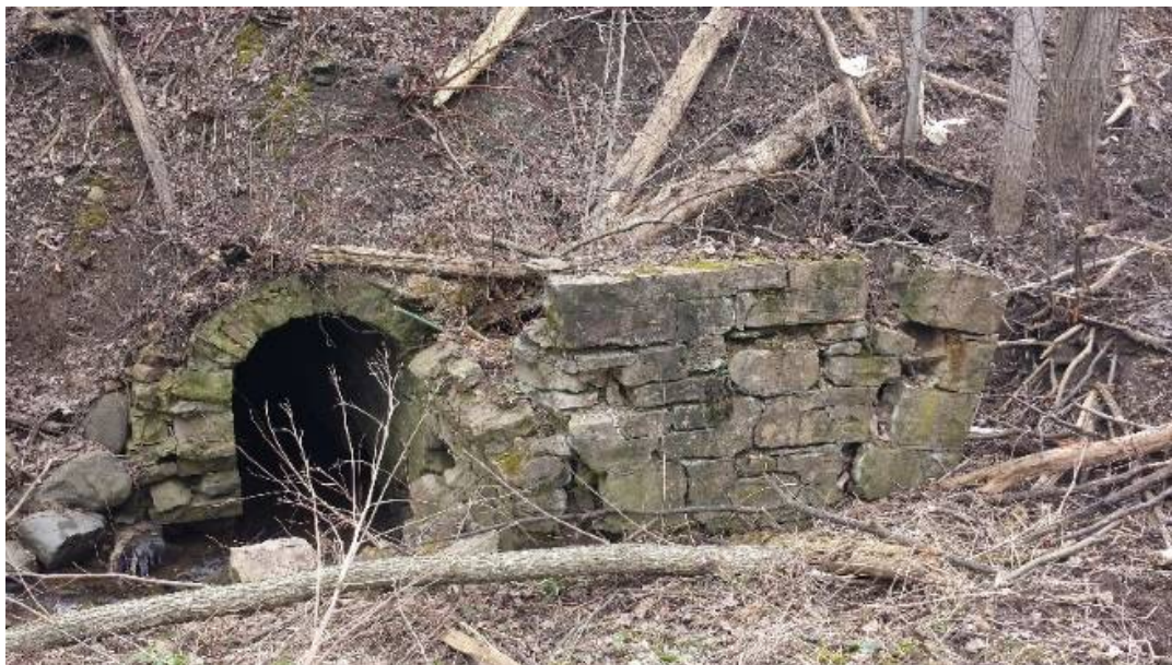
Figure 3 - Culvert inlet pre-construction
