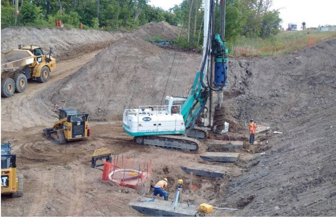
Figure 10 – Construction of roadway shoring with access to valley completed
