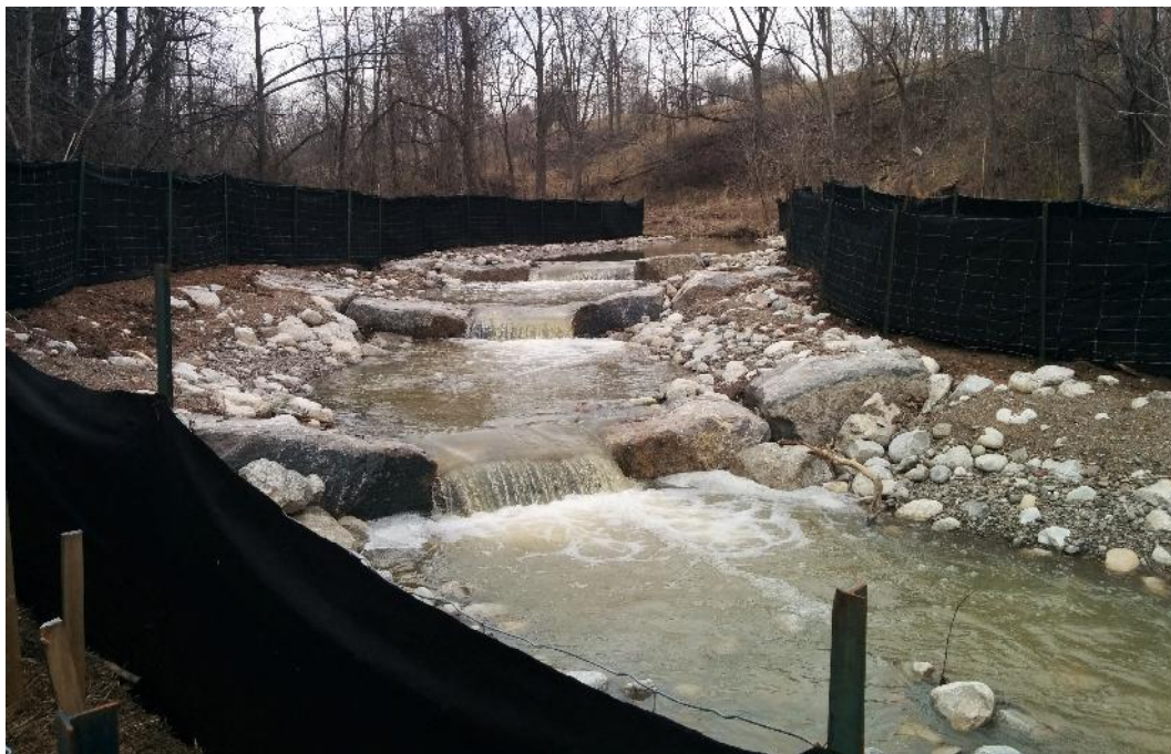
Figure 7 – Completed pool-step transition
