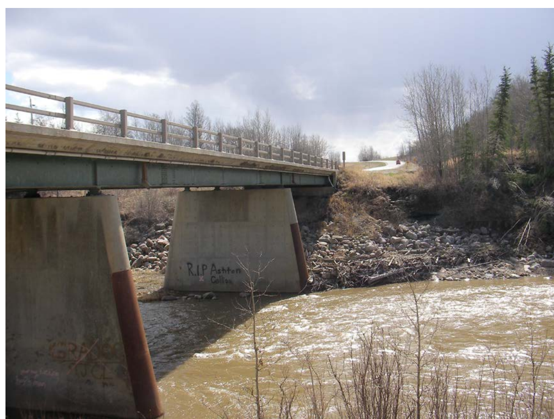
The 3-span bridge over Redwillow River
