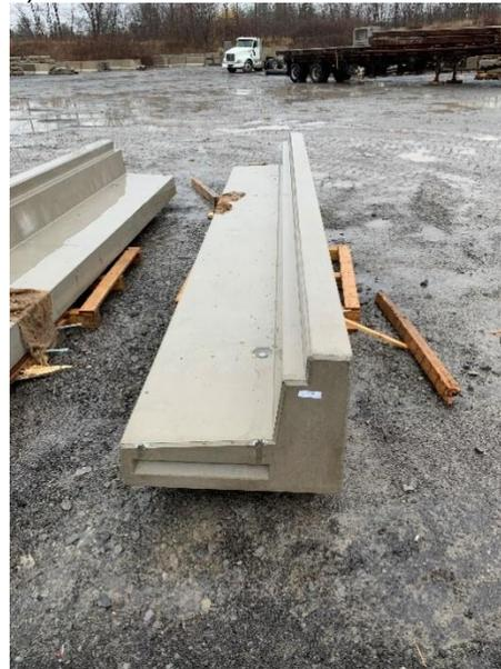
Figure 6 - Curbs designed for the corridor replacement program: a) 3D isometric view and; b) picture of a precast curb
