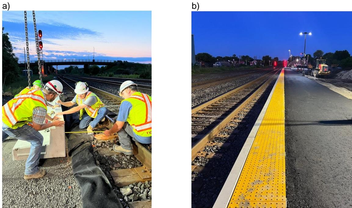
Figure 8 - Installation of a precast curb along the track.
