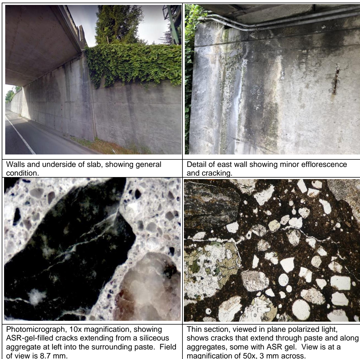
Figure 6: 65-year-old overpass concrete with minor ASR damage allowing continued serviceability.
