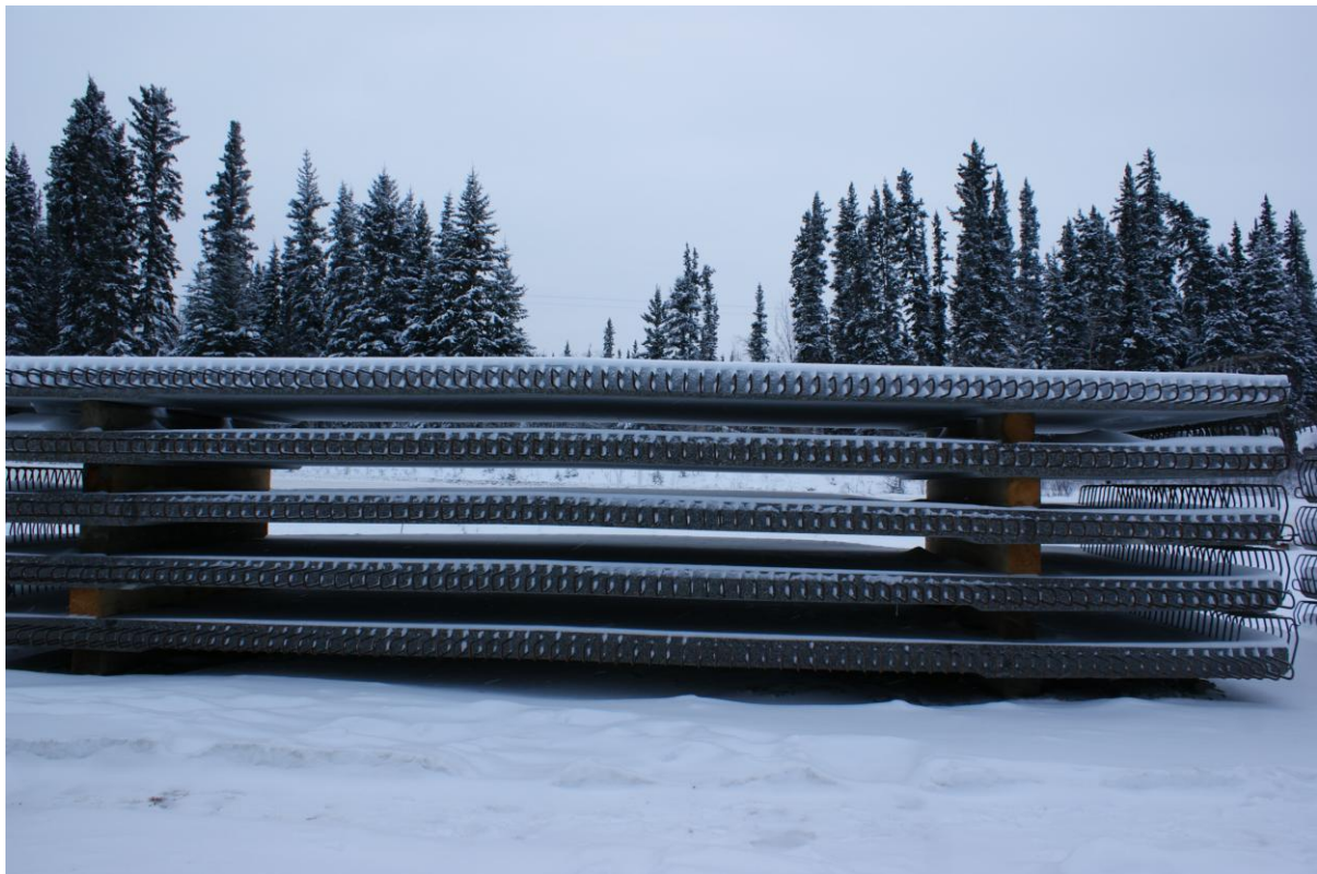
Fig. 9: Precast deck panels stored onsite (Photo: Arndt Becker, Infinity)
