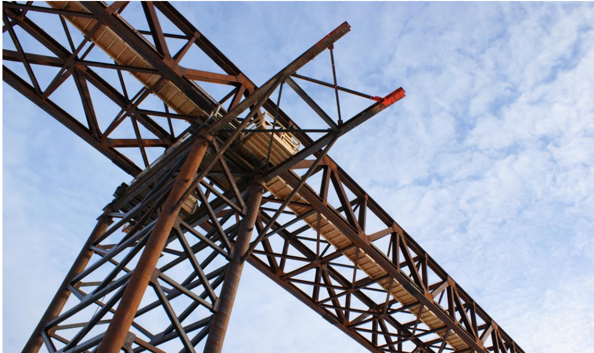
Fig. 10: Truss supported by the tallest temporary bent in the main span (Photo: Arndt Becker, Infinity)
