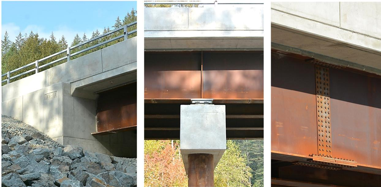
*Figure 4: Structural Details of the Chehalis Bridge: Integral abutment/girder connection (left), girder support at pier (middle), and bolted girder field splice (right).*
