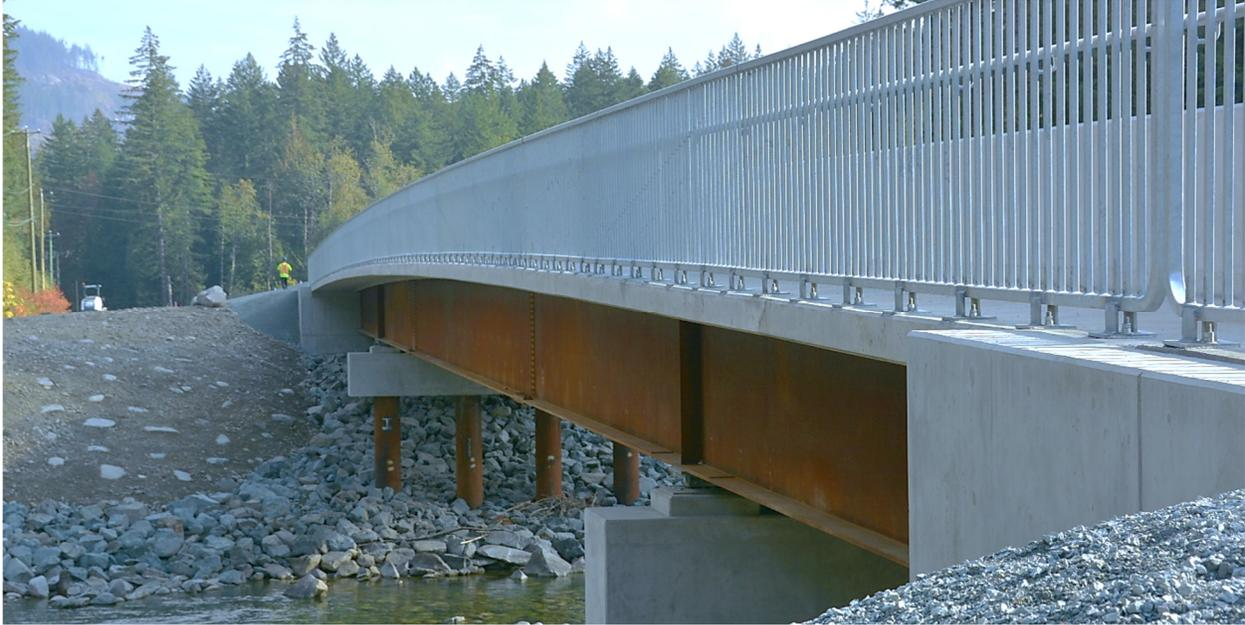
*Figure 6: Upstream side of the Chehalis Bridge showing the symmetrically hogged roadway profile and the direct load path from the girders into the piles.*
