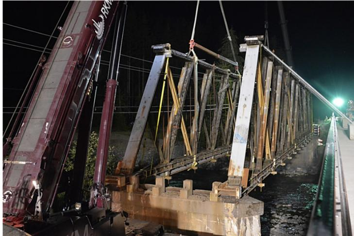
*Figure 14: Old Chehalis Bridge: Top chord of truss next to the new bridge (near side truss) stabilized with inclined struts which use the new bridge as anchorage.*
