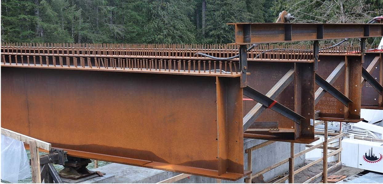
*Figure 10: Released mobile crane support after landing onto the rollers installed at the southern pier.*
