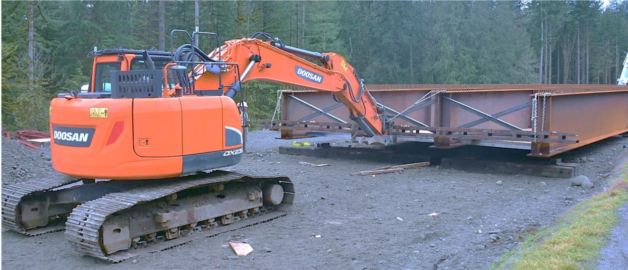
*Figure 7: Pushing excavator behind the northern abutment to facilitate incremental launching.*
