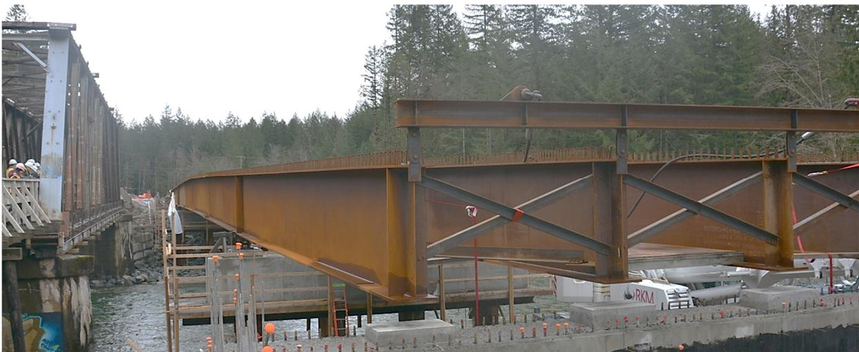
*Figure 11: Girders in their final position after the last push was executed.*
