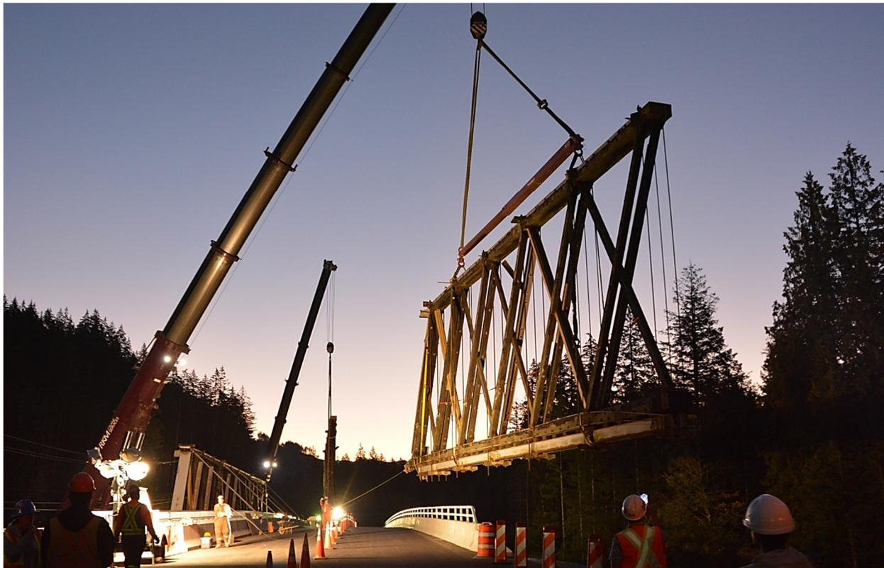
*Figure 18: Old Chehalis Bridge: Swing operation to guide the first truss half of the far side truss to the designated break-down location behind the abutment. In the background, the second half is still sitting on the new bridge before lifted to the second break-down area behind the opposite abutment.*
