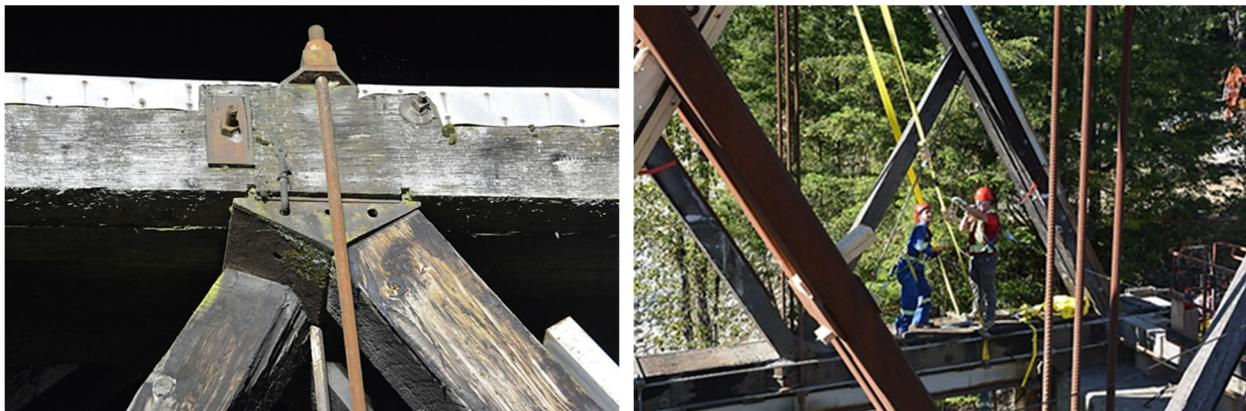
*Figure 15: Old Chehalis Bridge: Post-tensioned top chord node to maintain compression in truss diagonals (left) and temporary straps to ensure truss integrity in critical nodes during the lift (right).*
