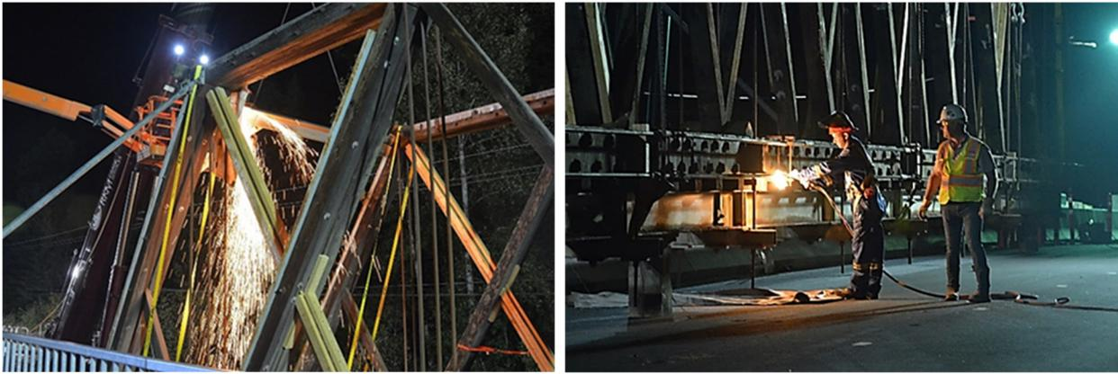
*Figure 16: Old Chehalis Bridge: Cutting the top beam of the end portal (left) and cutting the bottom chord in midspan while the truss is resting on the new bridge (right).*
