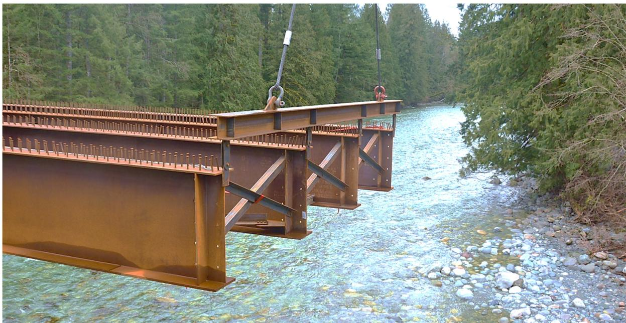
*Figure 9: Girder tip support via spreader beam and mobile crane in the main span.*
