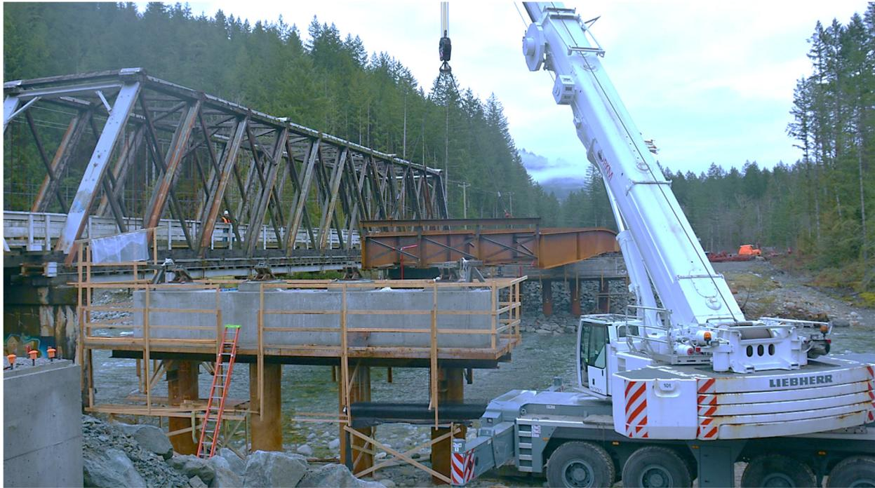
*Figure 8: Assisting mobile crane reduces the maximum cantilever moments and ensuring girders safely land of the rollers installed on the southern pier.*
