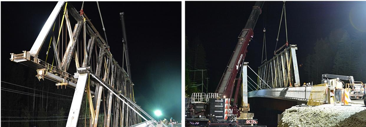
*Figure 17: Old Chehalis Bridge: Far side truss is lifted as one piece by two mobile cranes onto the new bridge.*
