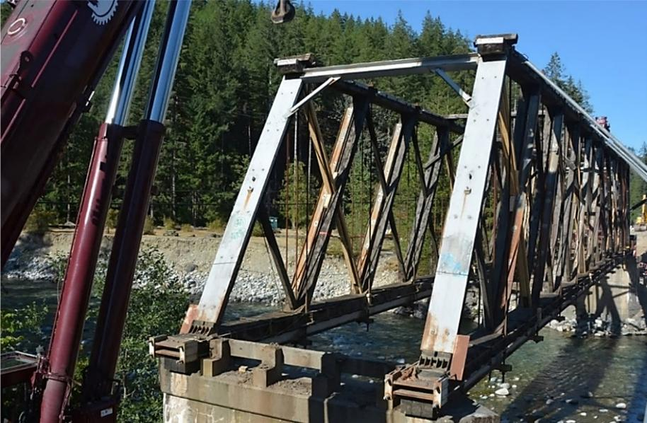
Figure 13: Old Chehalis Bridge: Naked truss structure with minimal lateral bracing components remaining at the day of removal.
