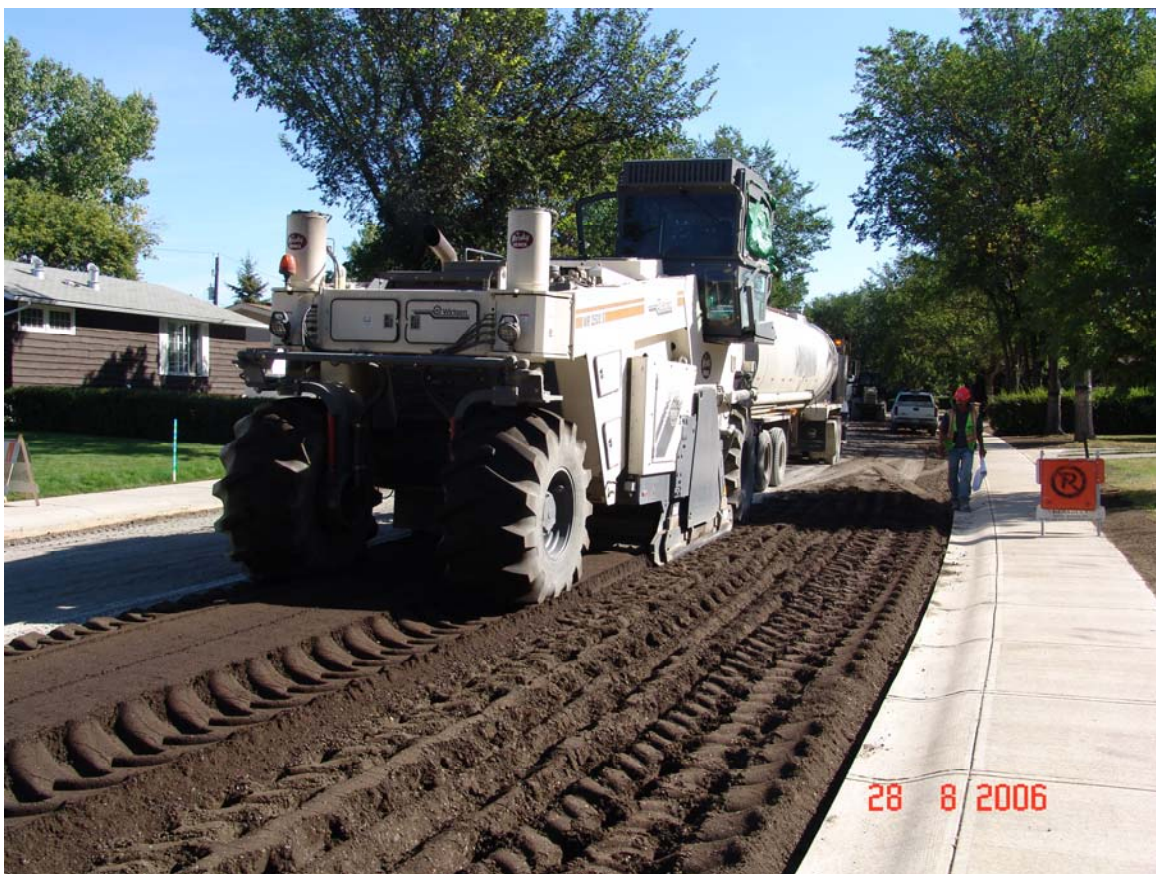
Figure 4.5 Cold In-Place Recycling and Feedback Stabilization Control System
