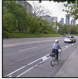
**Buffered Bicycle Lanes:** A buffered bicycle lane is marked primarily with white pavement markings running parallel to the roadway, that act as a buffer to increase the separation between bicyclists and adjacent motor vehicles.
