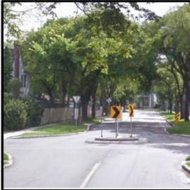
**Bicycle Boulevards:** Often located on local roads, bicycle boulevards incorporate traffic calming measures to facilitate through access by bicycles while inhibiting through access by motor vehicles
