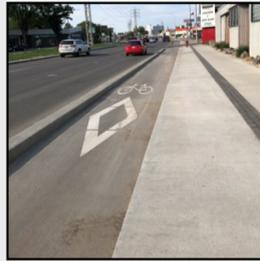
**Protected bicycle lanes or cycle tracks:** A protected bicycle lane is an on-road bicycle lane separated from motor vehicle traffic by a physical element, such as a curb.
