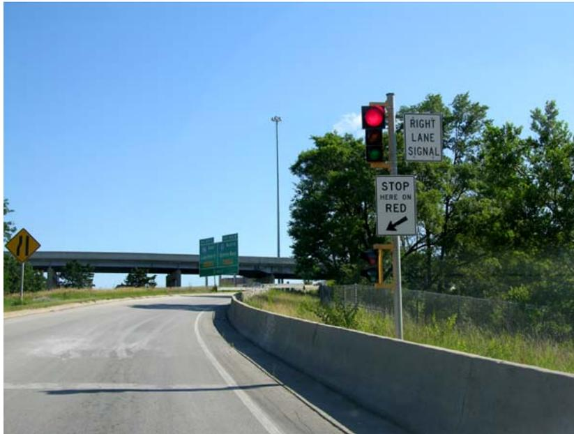
**Figure 5-3 – Ramp meter installed in Milwaukee, Wisconsin**
