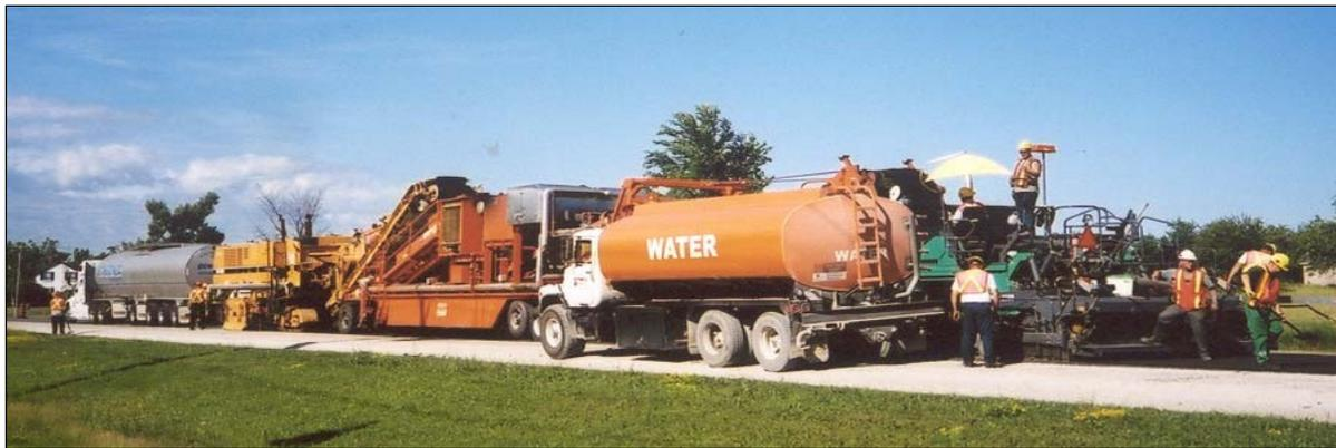
**Figure 3. Cold-In-Place Recycled Expanded Asphalt Mix Train**
