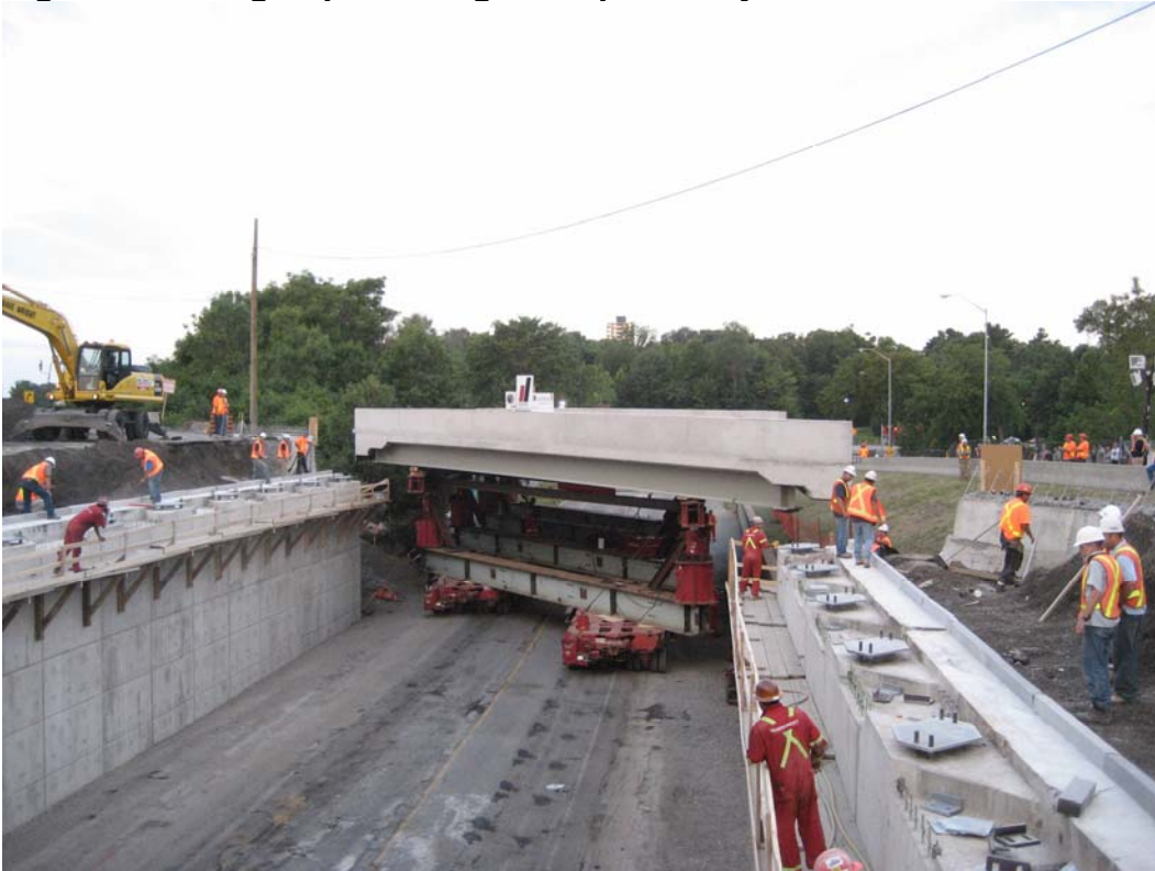
Figure 8 – Bridge Span Being Transported by SPMT
