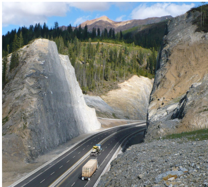
Figure 5 - 90 Metre Rock Cut on Kicking Horse Canyon Project (BC MoTI Photo)
