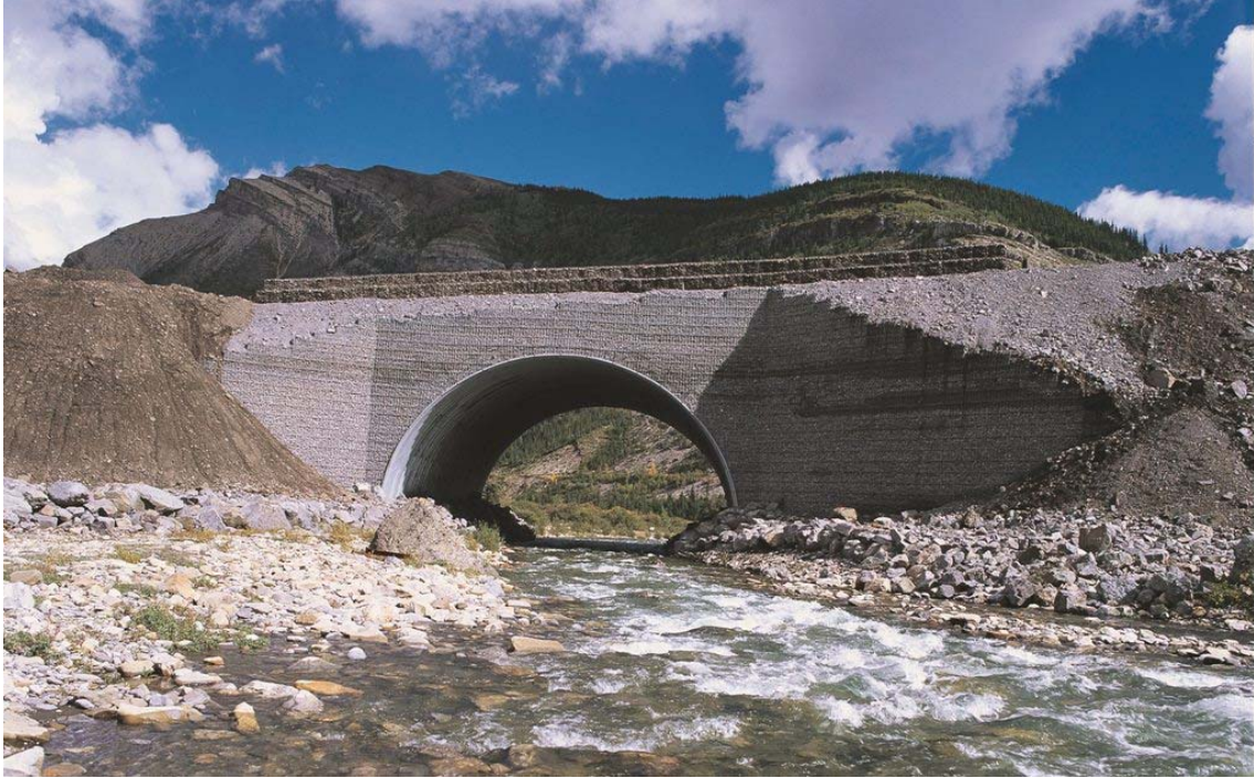
Figure 1. Whitehorse Creek Soil-Steel Arch Structure
