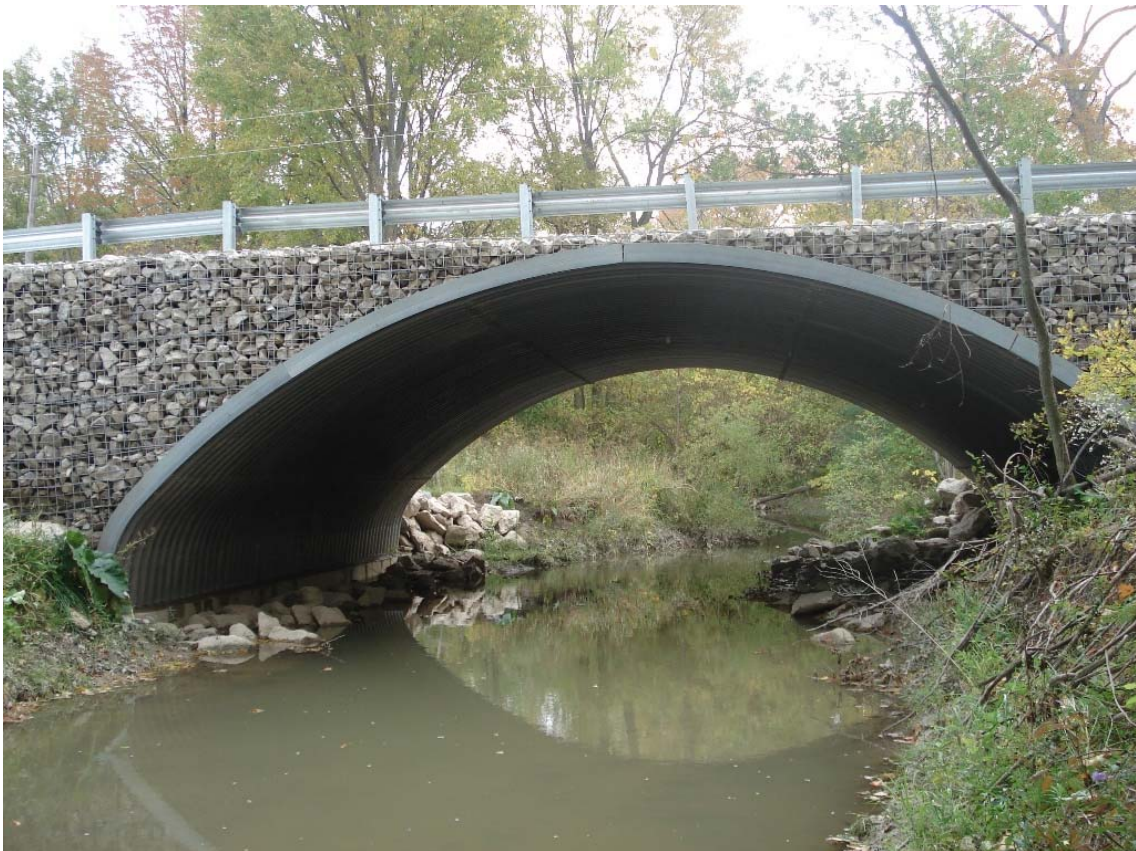
Figure 2. Aluminum Metal Box Structure
