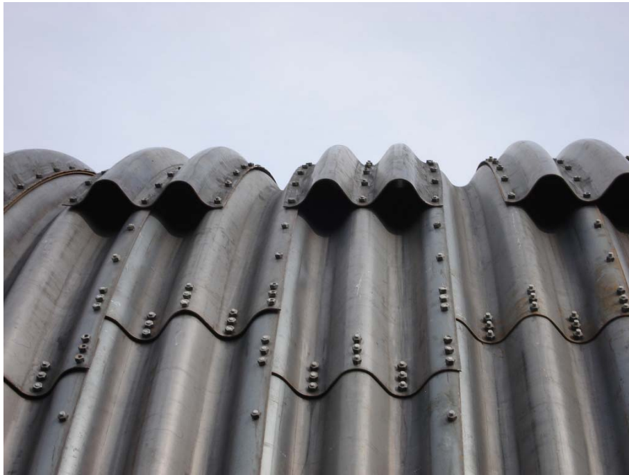
Figure 9. Steel arch with deep corrugated plate stiffeners on crown region
