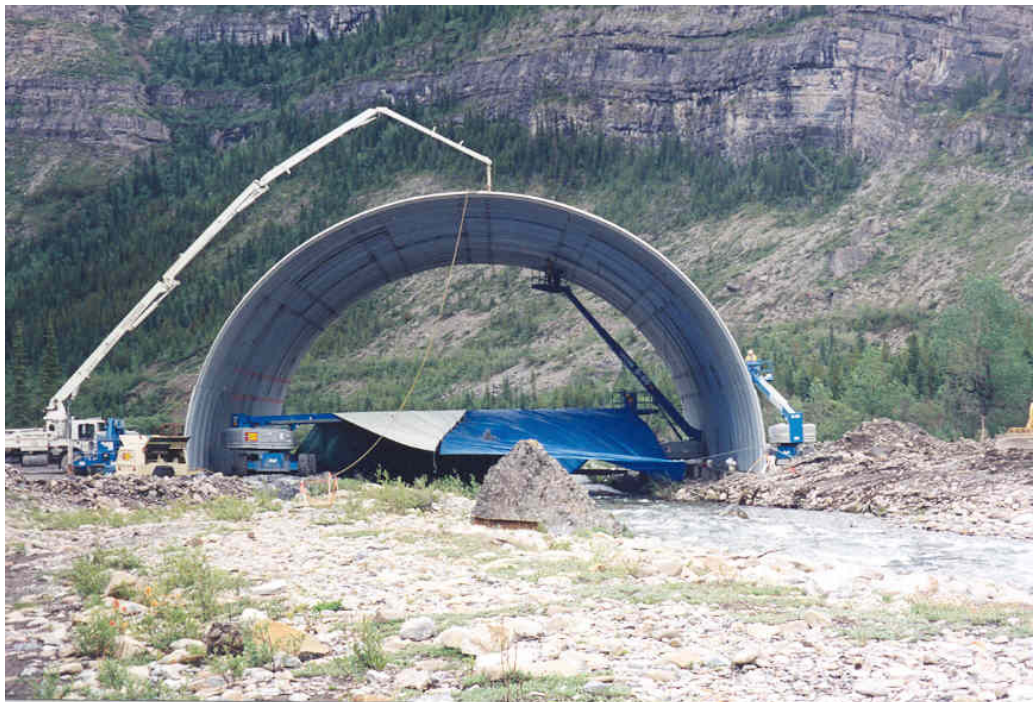
Figure 11. Concrete being pumped into voids between corrugated plates
