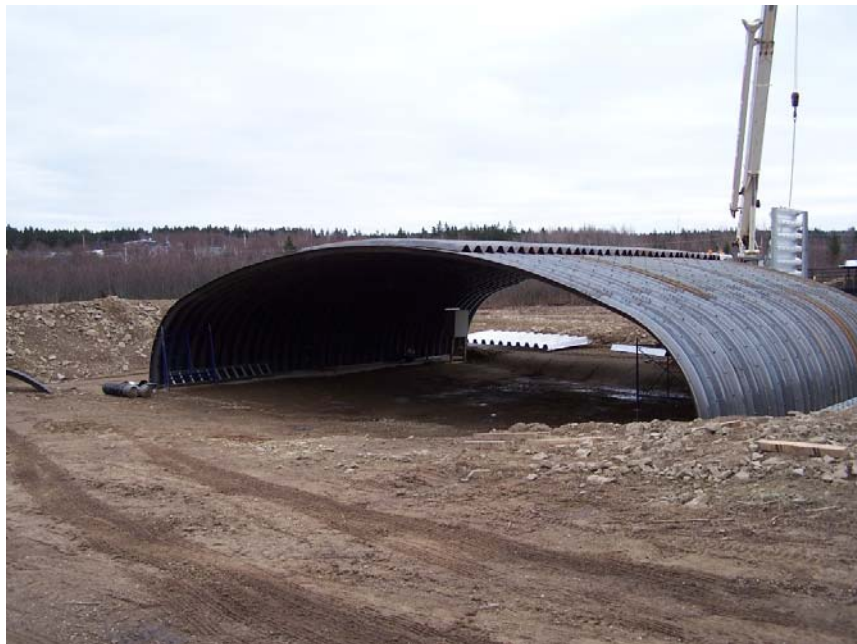
Figure 15. Construction of metal box test structure in Dorchester, New Brunswick
