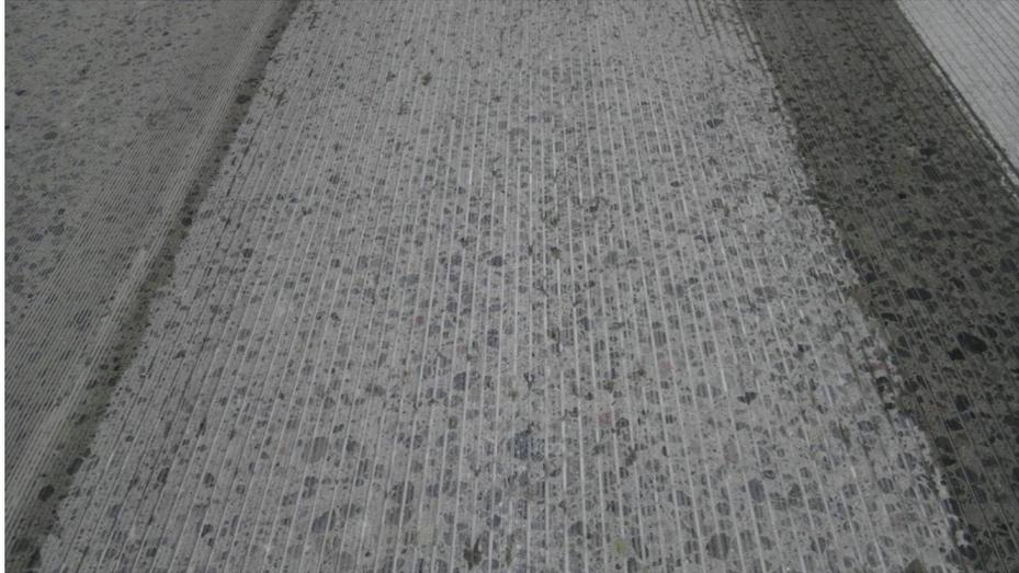
**Figure 2. Newly Longitudinally Grooved Concrete Pavement on Highway 115**
