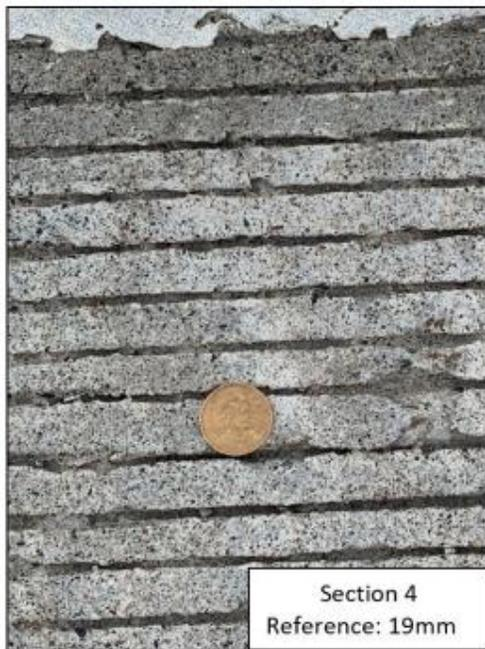
Concrete – Longitudinally tined
