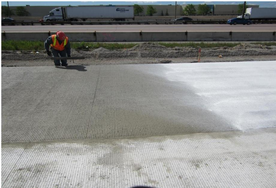
**Figure 3. Concrete Pavement with Transverse Tining on Highway 401**
