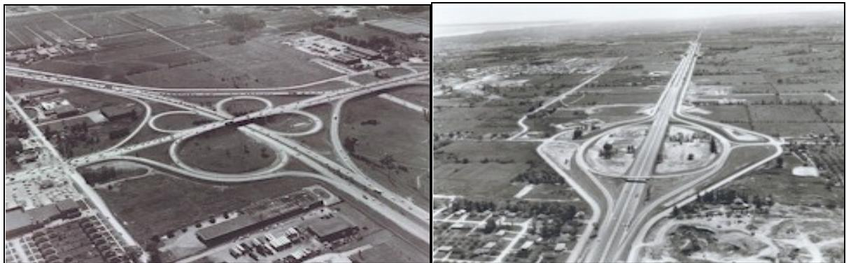
Figure 2 – Cloverleaf and Diamond/Traffic Circle Interchanges on the QEW, 1937-1940
