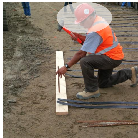
Figure 7: Preparing lumber for tensioning of reinforcement
