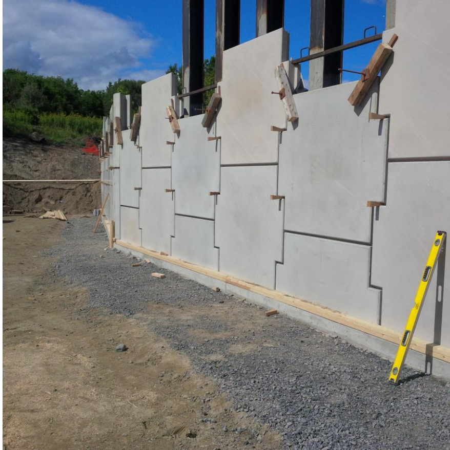
Figure 11: Hurdman East Overpass under construction
