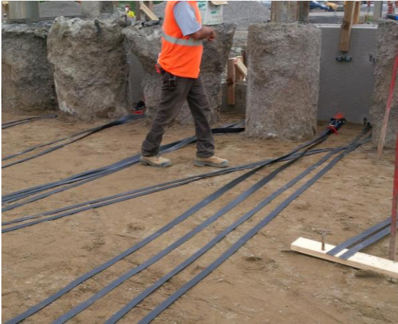
Figure 10: Reinforcement being skewed past obstructions
