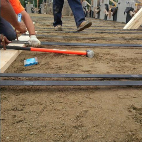
Figure 9: Tensioning soil reinforcement
