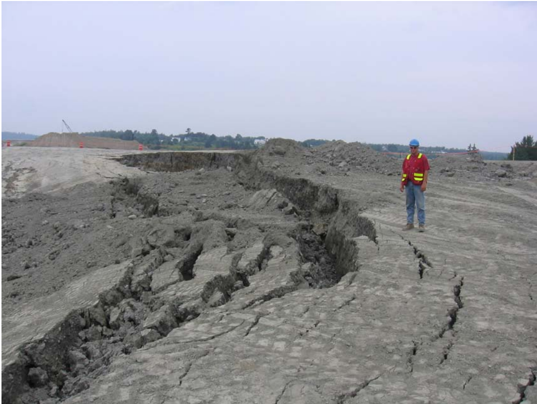
Figure 1: Embankment Failure
