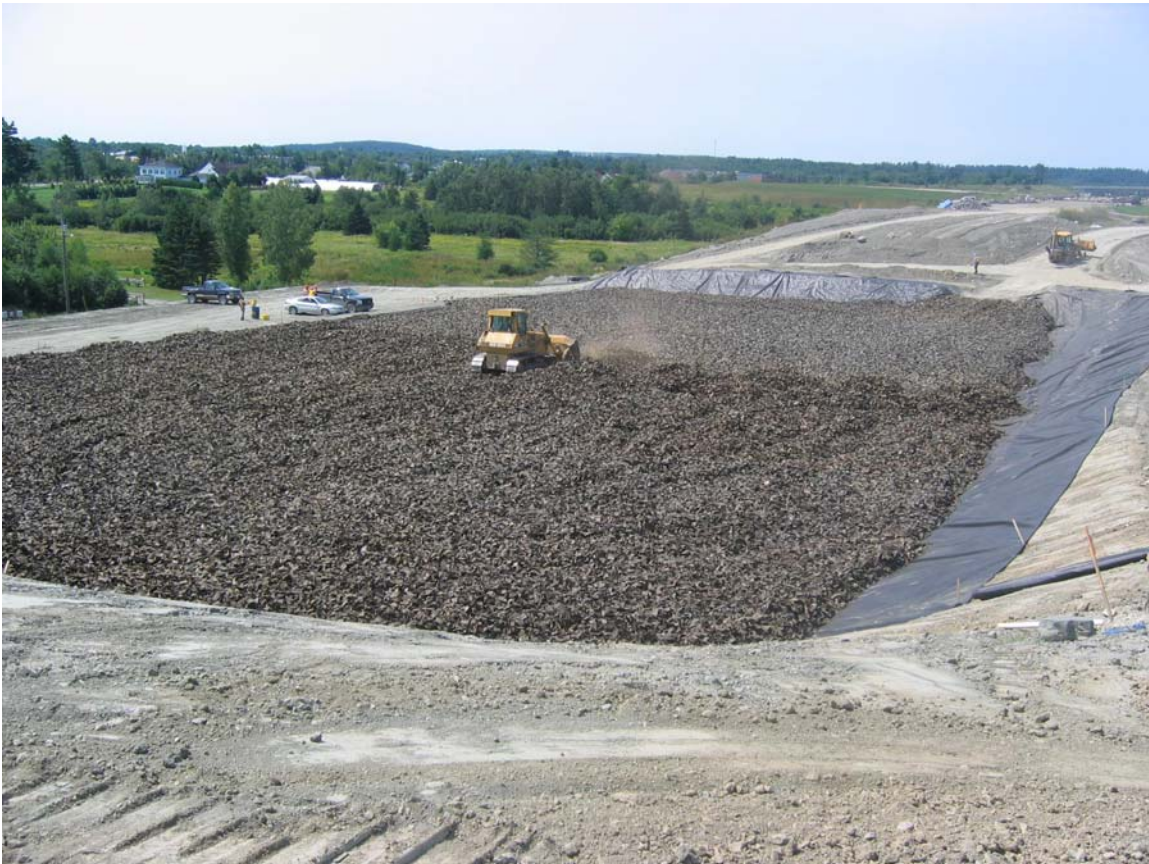
Figure 4: Spreading TDA with a bulldozer
