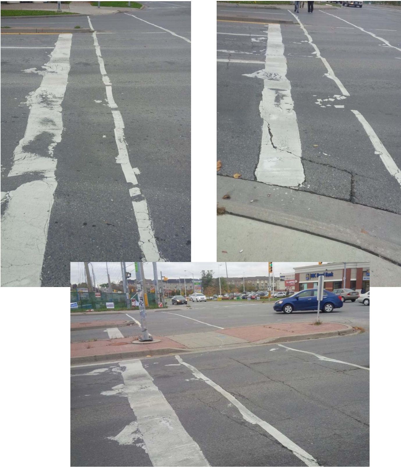
Figure 1 – Asphalt distresses at the intersection approaches (photos from 2014)
