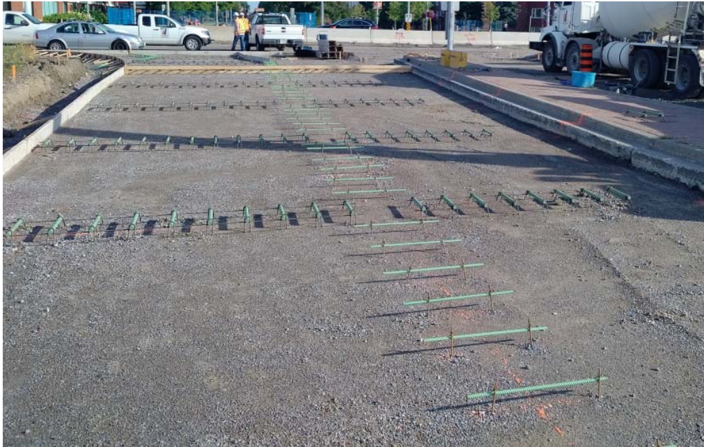
Figure 4 - Dowel baskets and tie bars in place
