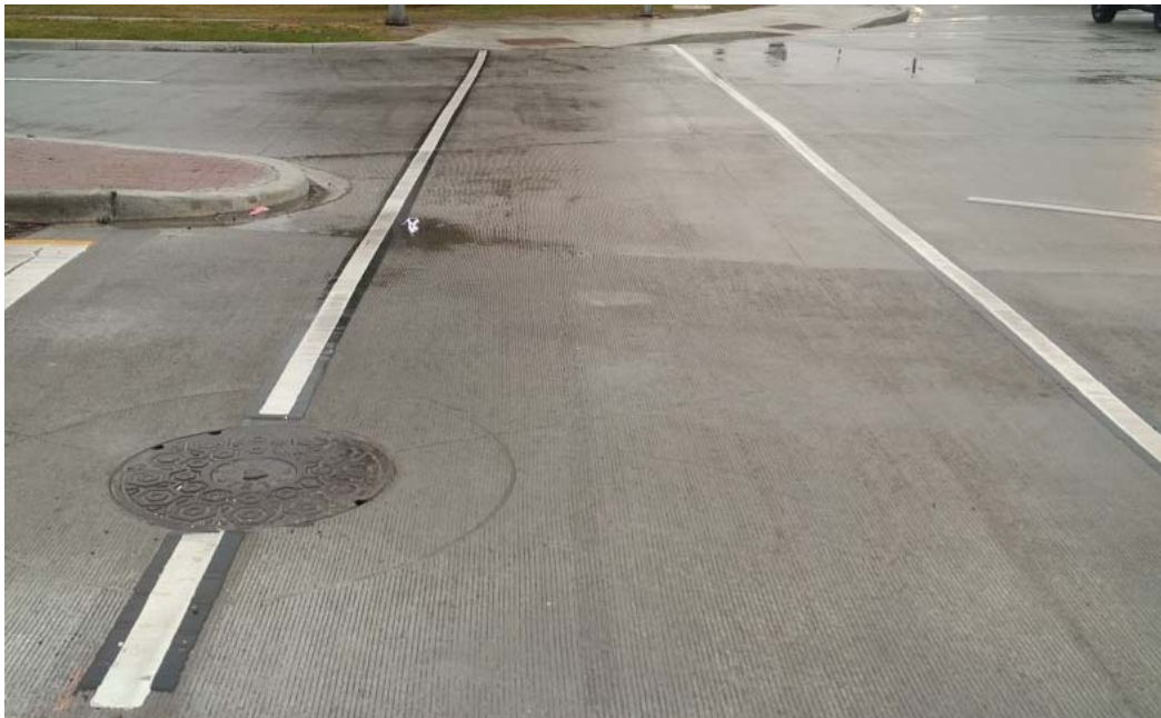
Figure 5 - Methyl methacrylate pavement markings with black backing on new concrete
