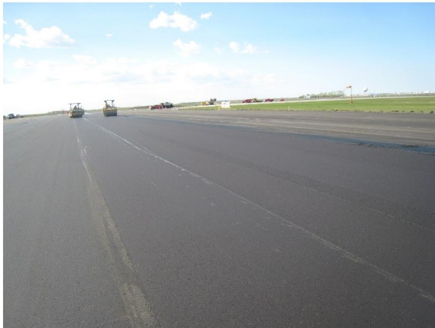
Photograph 19: Excellent quality of surface course mat. Longitudinal joint is very tight.
