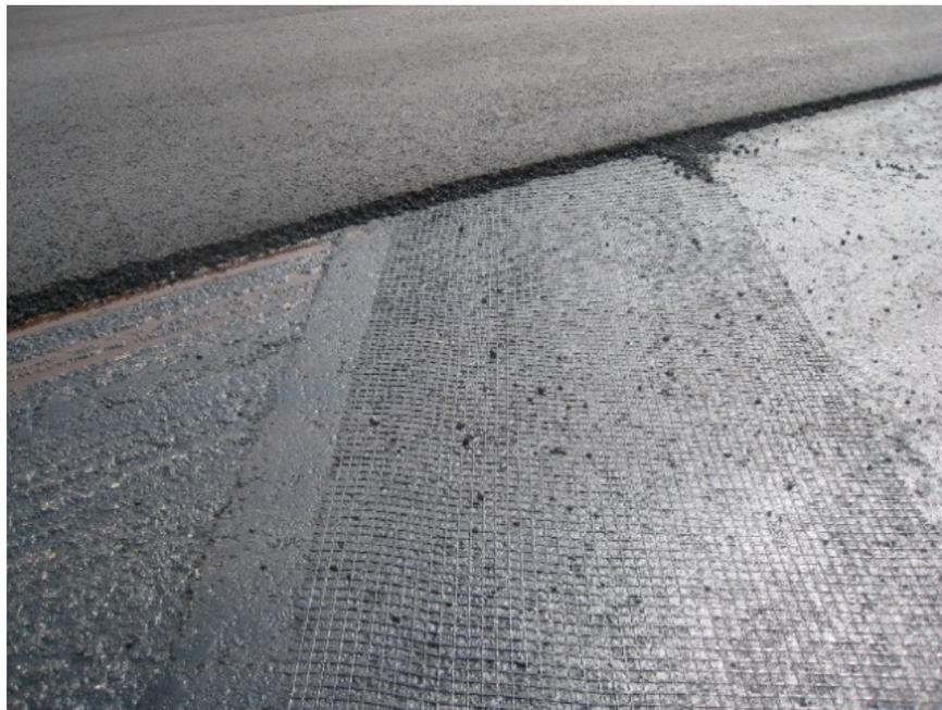
Photograph 17: GlasGrid® placed on existing pavement below the lower course.
