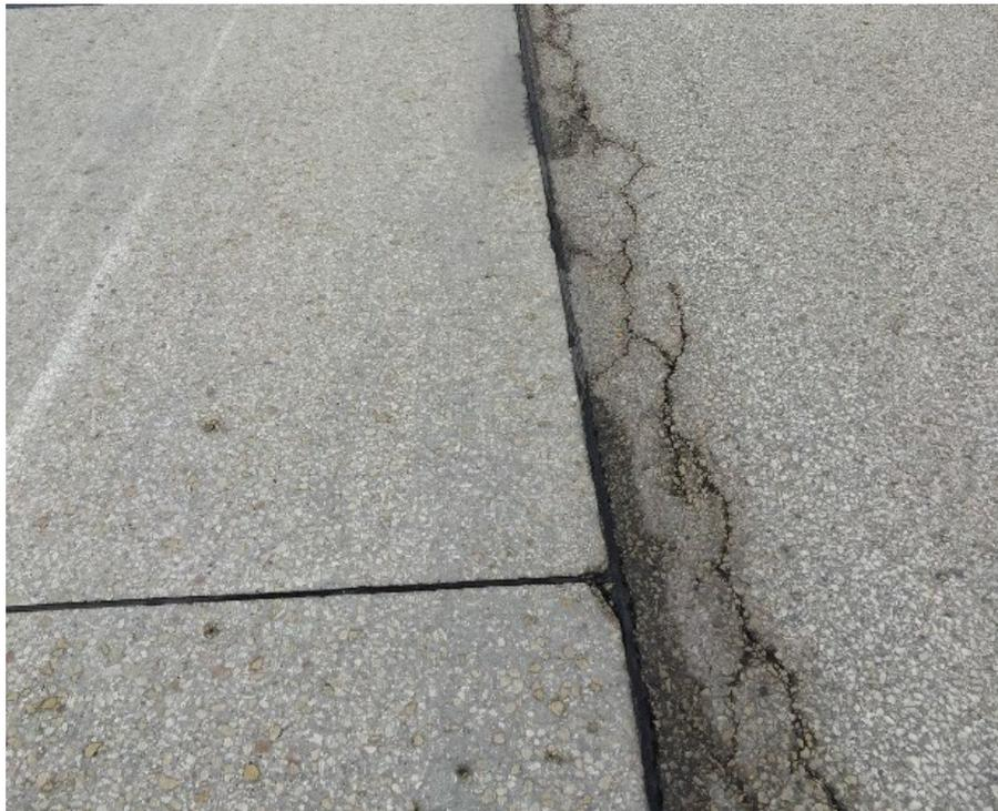
Photograph 12: Severe longitudinal crack along the concrete/asphalt interface.
