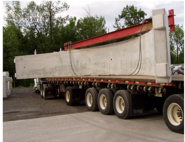
**Figure 4. Moving Arch to Storage Yard**
