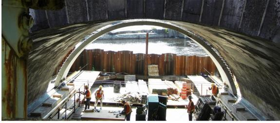
**Figure 8. Pulling First Arch Segment into Arch 1**
