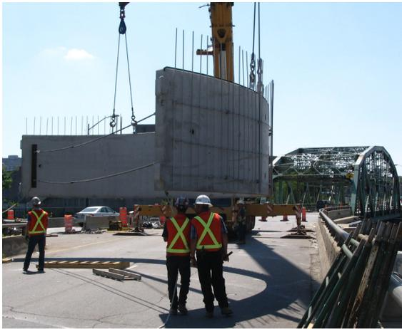
**Figure 5. Leapfrogging of Crane and Arch into Position**
