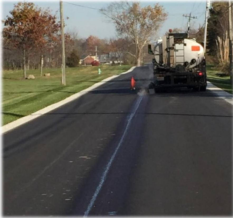
**Figure 4: Joint Sealer being applied by a distributor over the LJ after both lanes have been placed.**
