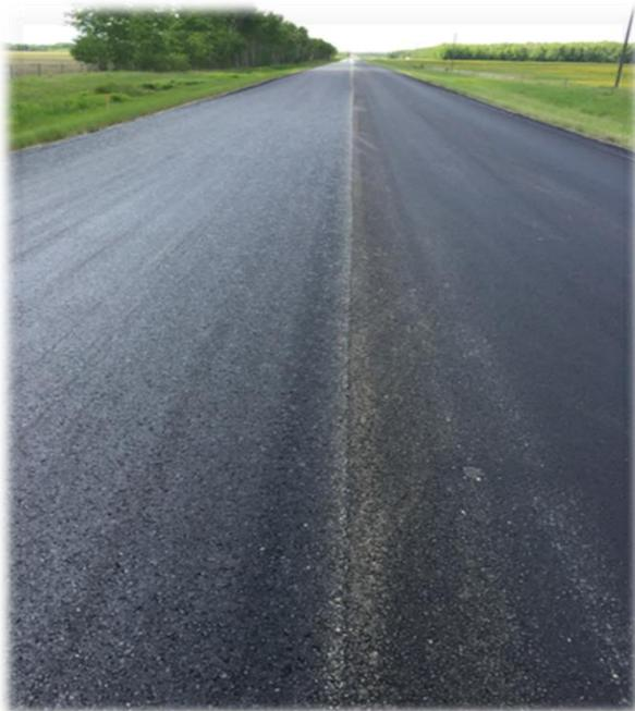
a. Newly constructed; uniform appearance, tack coat applied to the interface.
