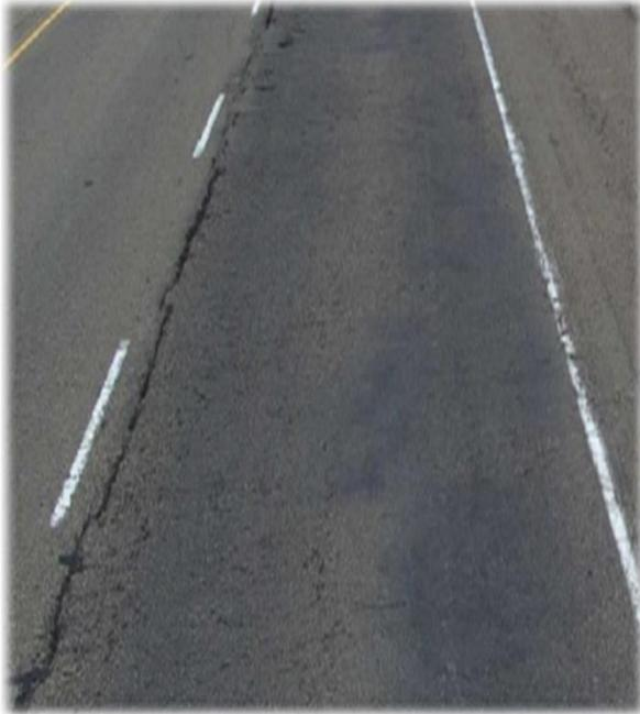
c. 8-year-old LJ with cracking and some spalling
