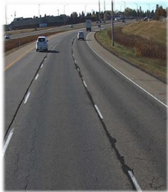
d. 14-year-old LJ previously repaired that is cracking and spalling
