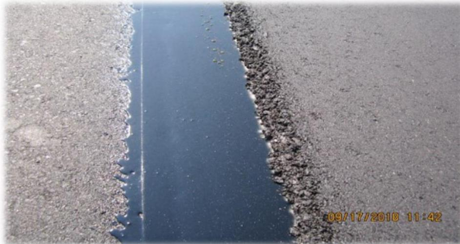
**Figure 7: Application of joint adhesive (VRAM) prior to placing a surface layer of asphalt.**
