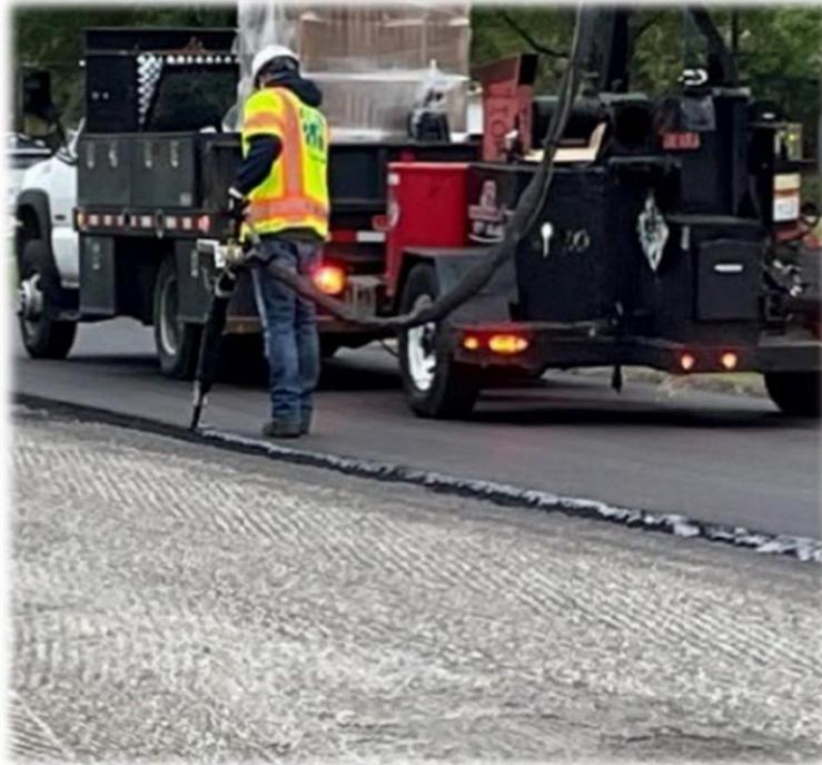
**Figure 6: Application of Joint Sealant to the face of the first pass.**
