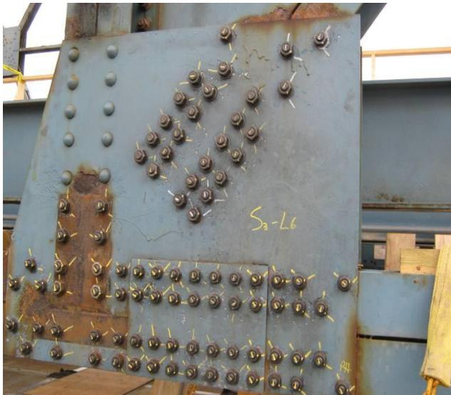
Figure 3: Rivets replaced by high-strength pretensioned bolts at all critical tension connections.
