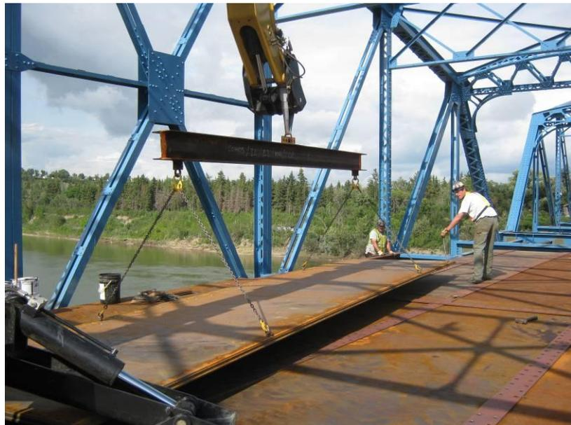
Figure 6: Installation of composite steel plate and elastomer decking panels.
