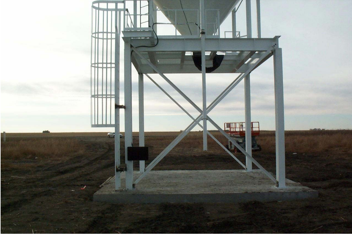
Figure 7 - Support Structure for a 90-tonne Salt Silo
