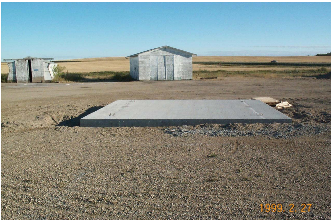
Figure 6 - Concrete Mat for 90-tonne Salt Silo at Meacham
