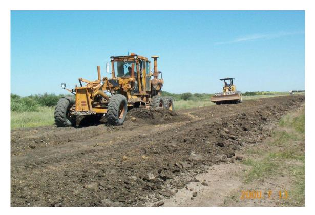
Figure 10 – Blading Off Geocomposite
