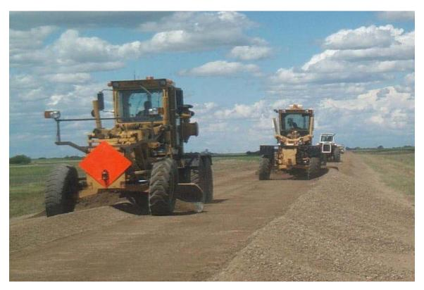
Figure 13 – Base Aggregate Overlay
