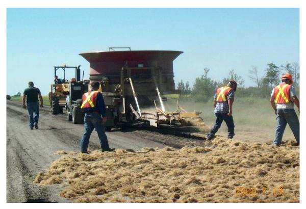
Figure 7 – Spreading of the Flax Straw Pieces
