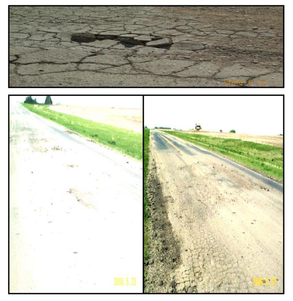
Figure 1 – Surface Failures on TMS Highway 19
