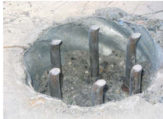
Figure 10 Stud Deformation
