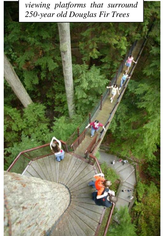
to the sensitive tree bark, or the delicate tissues beneath. Not a single saw-cut, bolt or nail into any tree was required to construct this design. We believe this to be a world first.
