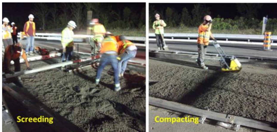
Figure 13: Compaction of the CTBM Grade Supported Slab Method
