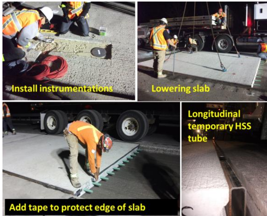
Figure 10: Precast Concrete Slab Installation (Asphalt Supported Slab)
