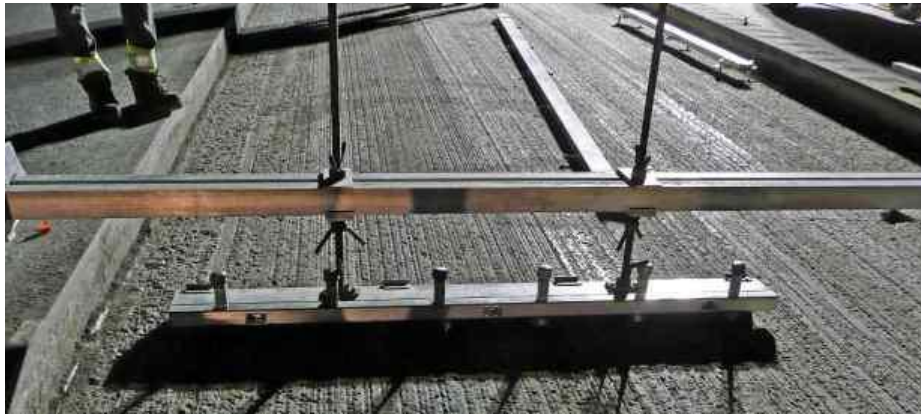
Figure 9: Fort Miller Grade Checker Apparatus
