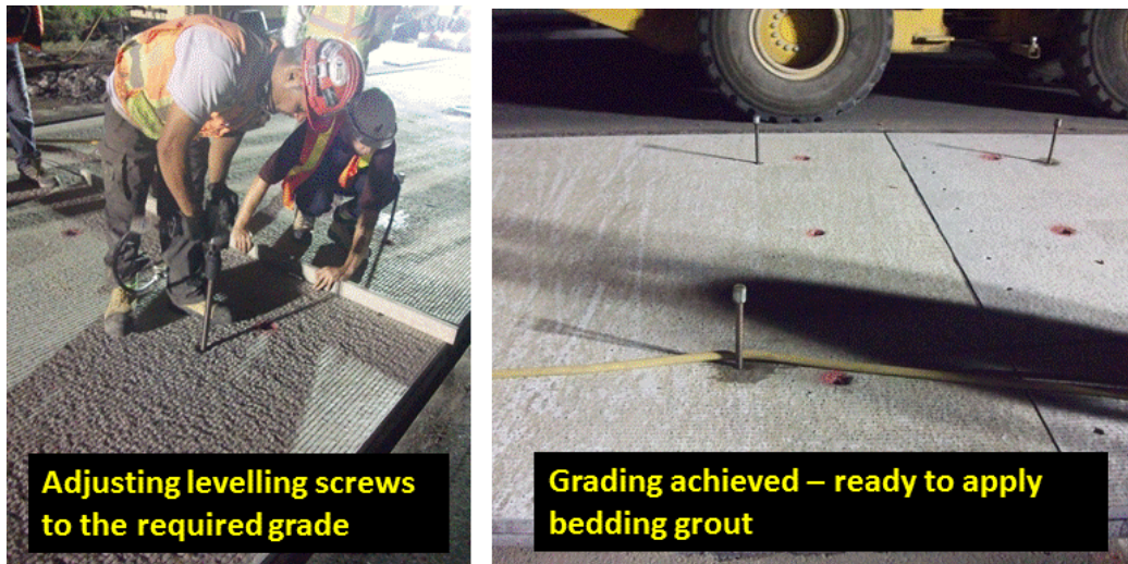
Figure 14: Grout Supported Slab Levelling Screw and Adjustment
