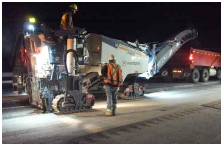
Figure 8: Wirtgen Milling Machine
