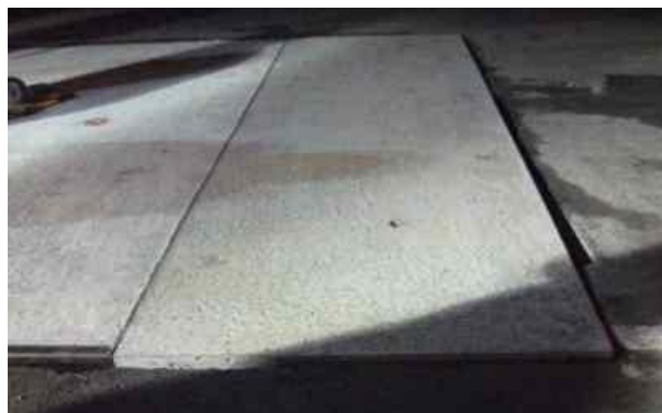
Figure 11: Asphalt Supported Slab and Temporary End Slab
