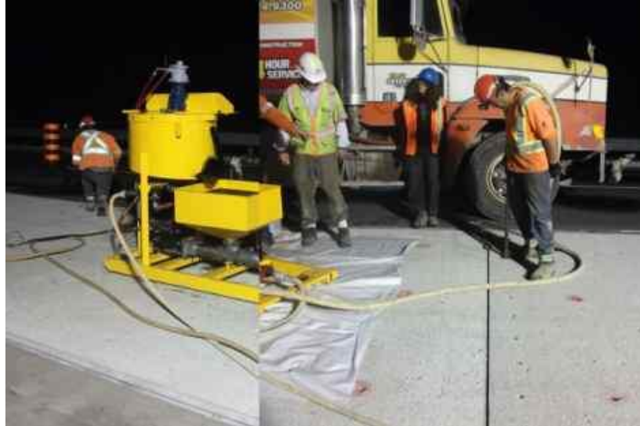
Figure 12: Pumping the Dowel Grout
