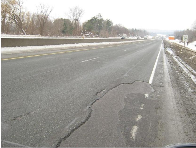
Figure 4: Delamination of DFC
