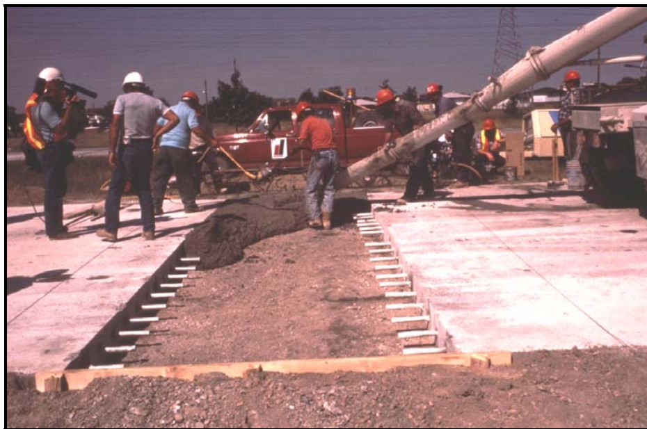
Figure 1. Typical Full Depth Repair in NBL
