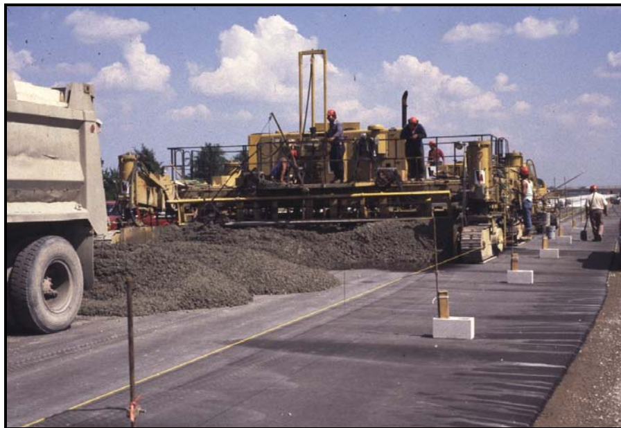
Figure 2. Slipforming Unbonded Concrete Overlay in SBL
