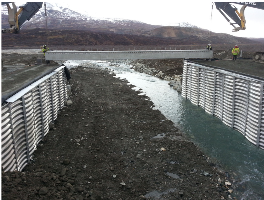
Figure 19: Girder Erection
