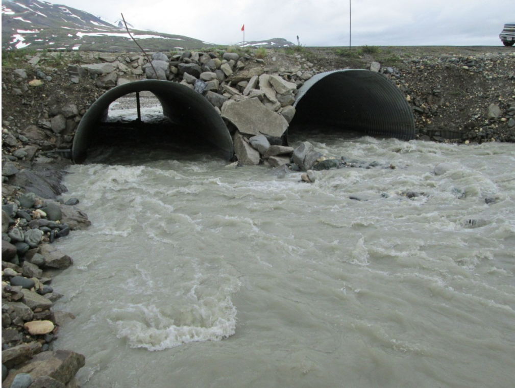
Figure 5: Spring 2013, Jack Posts in North Culvert, Embankment Settlement Over North Culvert
