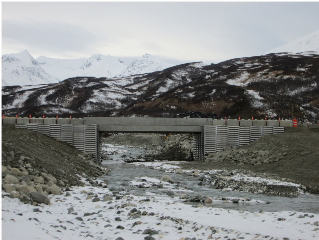
Figure 22: Completed GRS-IBS with Temporary Guiderails (view from downstream)
