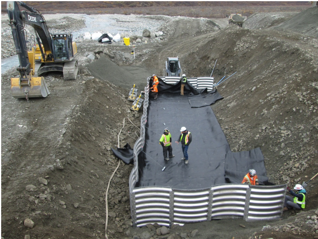
Figure 14: Construction of South Abutment
