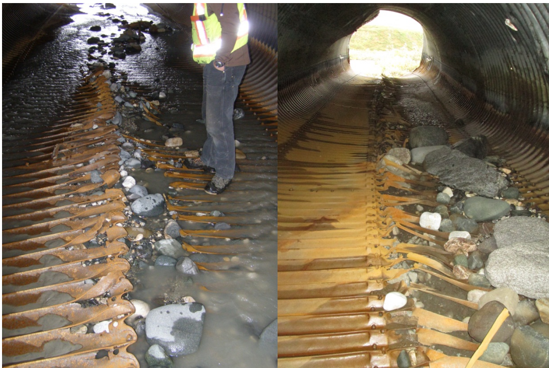
Figure 4: Abrasion Damage on Bottom of North (left) and South (right) Culverts
