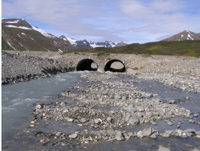
Figure 3: Fall 2012 Nadahini Creek Twin Structural Plate Pipe Arches (SPCSPA)
