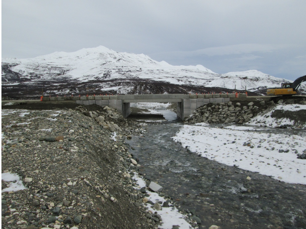
Figure 21: Completed GRS-IBS with Temporary Guiderails (view from upstream)
