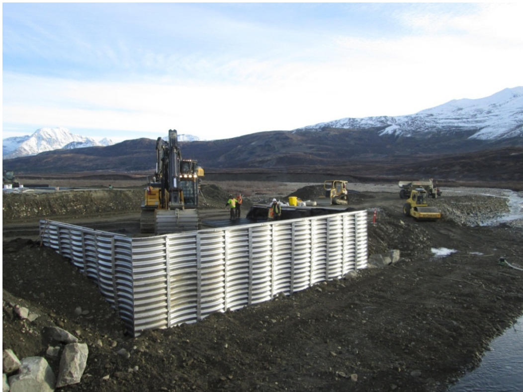
Figure 16: Construction of North Abutment
