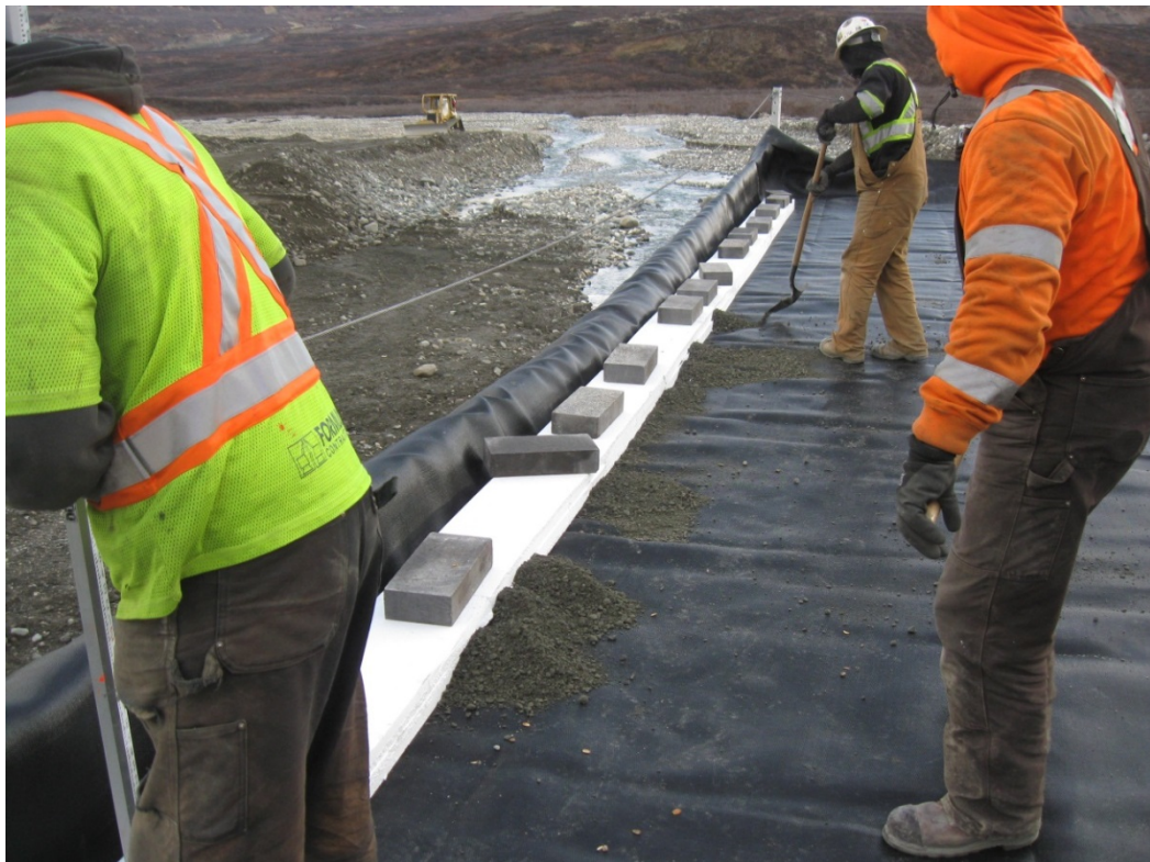
Figure 18: Placing foam board for beam seat zone
