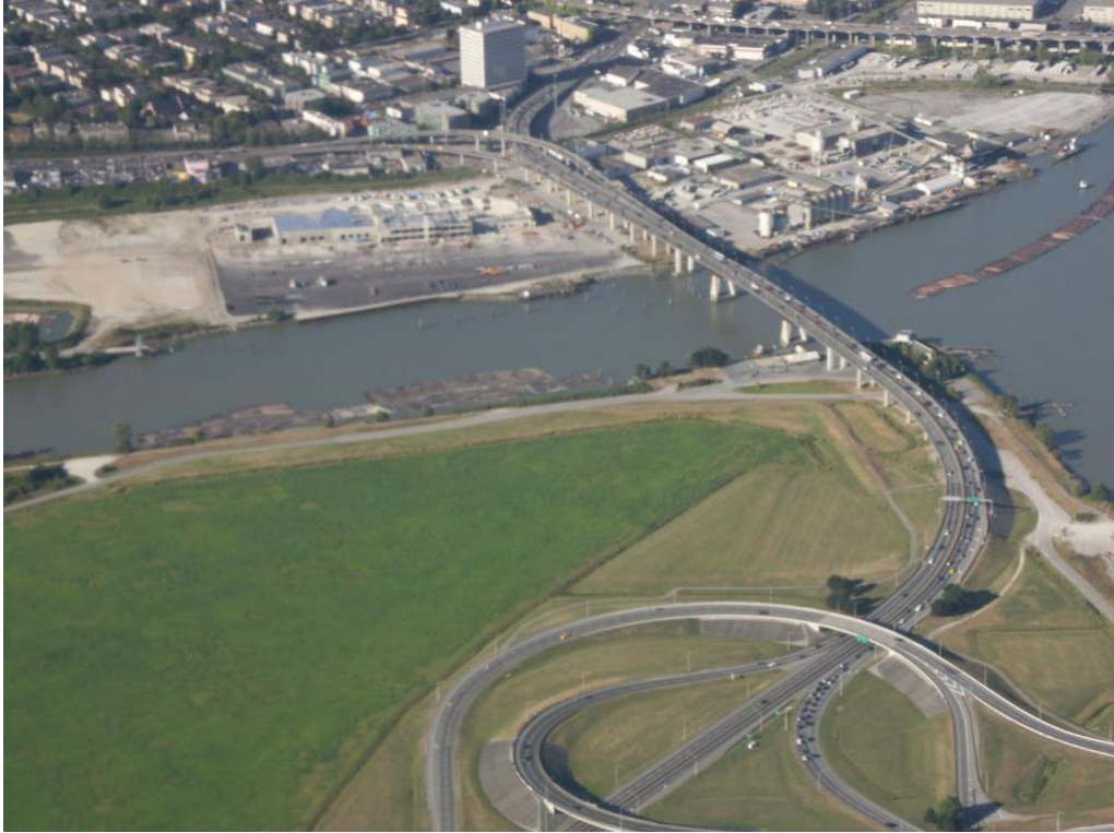
Figure 2: General view of the Bridge
