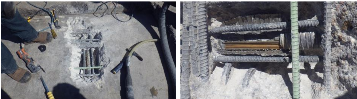
Figure 5 - Exposing Post-Tension Cable Duct
