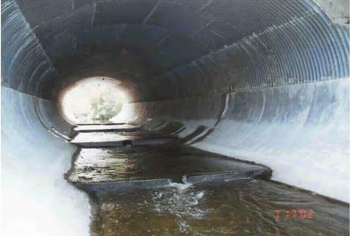
Figure 4 – Completion of Typical Rehabilitation
