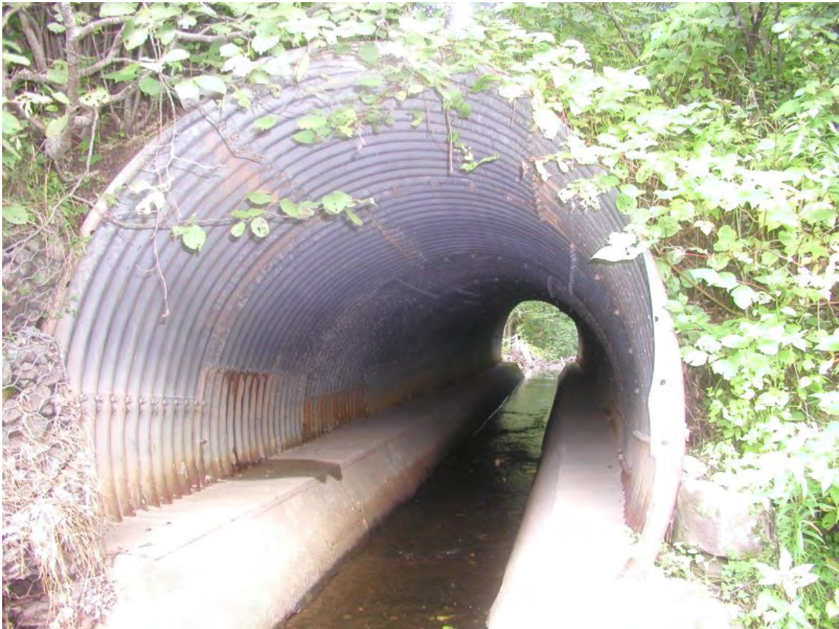
Figure 2: SPCSP Bridge Rehabilitated in 1987
