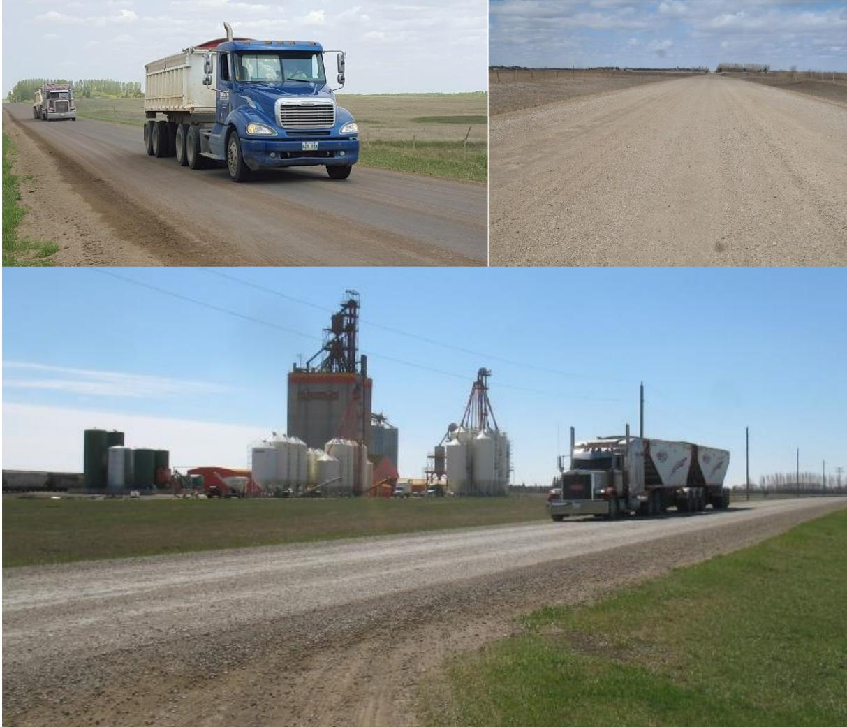
Figure 2: Curries Landing Road after stabilization in 2015 (top left), and in April 2020 (top right). Pioneer road after stabilization in 2018 (bottom).
