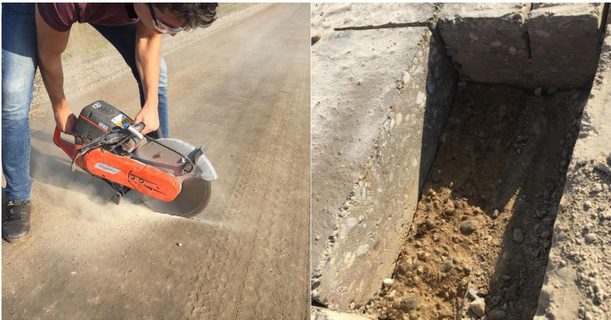
Figure 10: Lori Road after stabilization and reconstruction with a 15cm thick wearing surface of A-base aggregate plus Penner clay mixed to ~32% -200 mesh fines resulting in ~10% cohesive clay minerals in the final mix. Left) Zach Toews using a concrete saw to cut blocks for examination and testing. Right) Profile through Lori Road in 2018, 3 years after stabilization.
