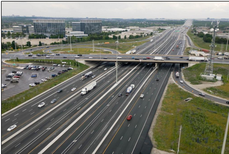
Figure 6: Completed widening of Highway 401
