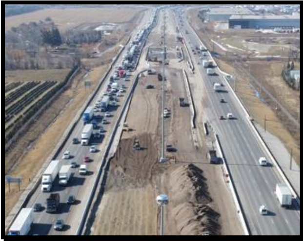
Figure 5: Traffic volume impact by direction
