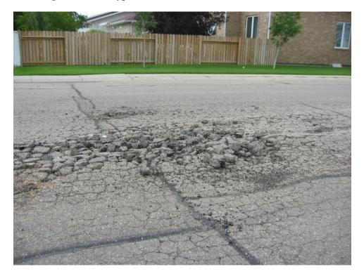
Figure 2Typical City of Saskatoon Roadway Structural Failure
