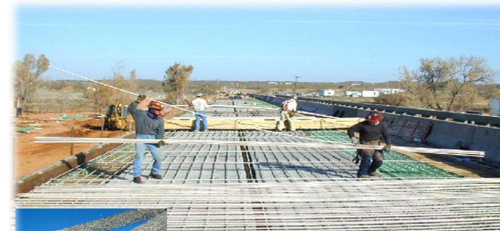
FRP application in RC bridge deck slabs
