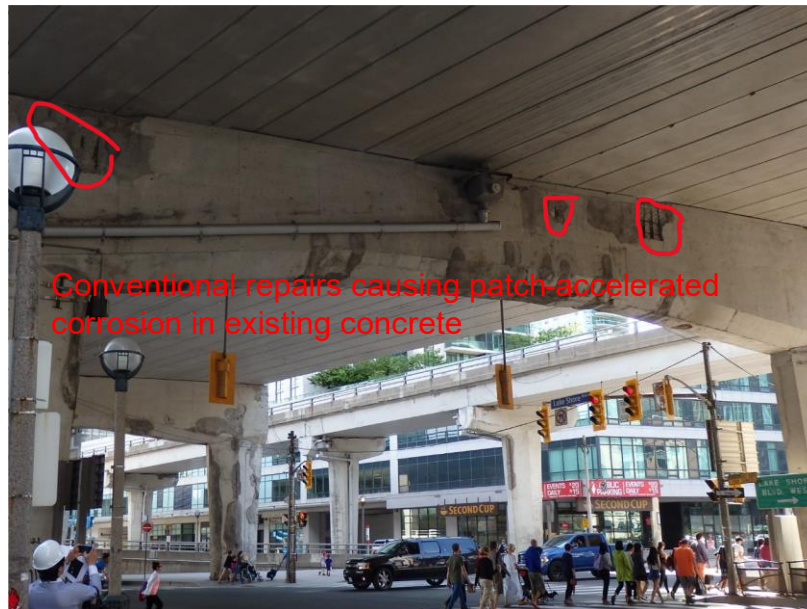
Figure 8. Patch-accelerated corrosion
