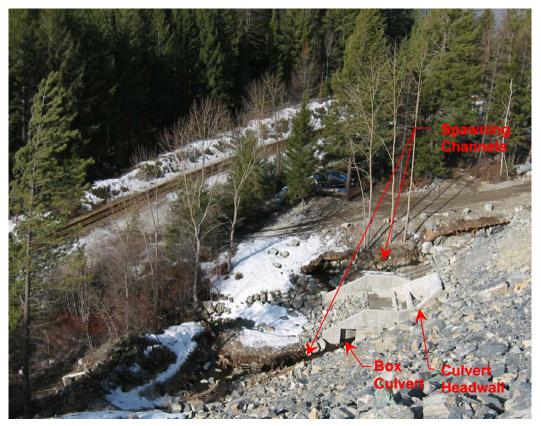
PHOTO 1 – SPAWNING CHANNELS AND CULVERT OUTLET
