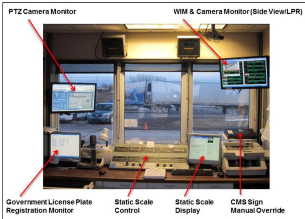
Figure 11 – Weigh Station Operations Center
