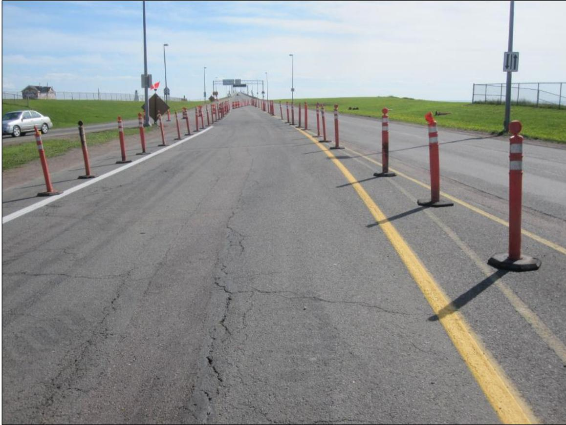
Figure 5 – Pavement before Resurfacing
