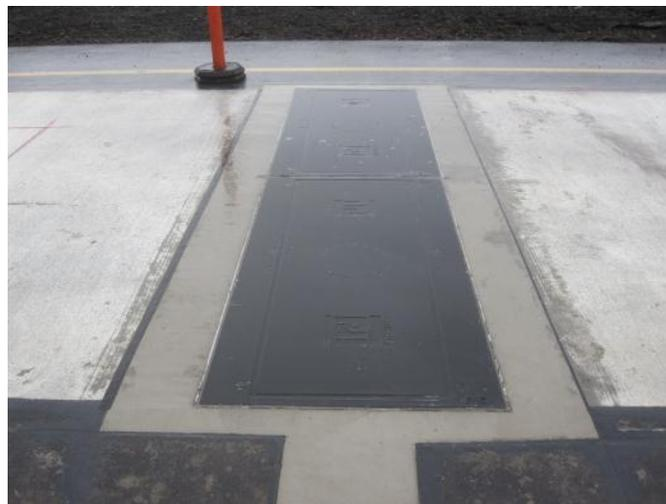
**Figure 9 – Single Load Cell (SLC) WIM**
