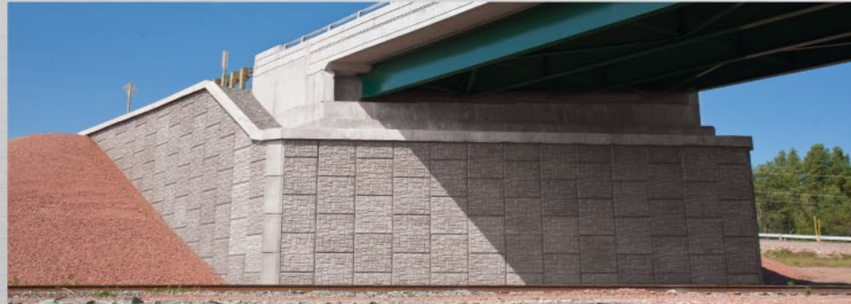
Figure 1. Completed Abutment, Spring Hill Junction, NS
