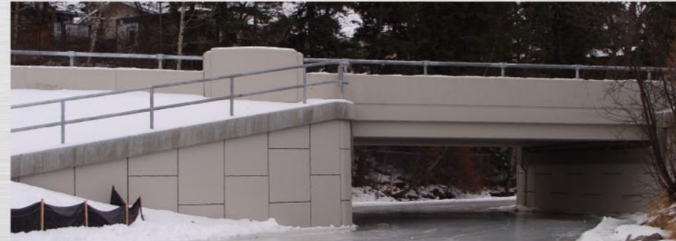
Figure 2. Completed Abutments, Bowness Park, Calgary, AB
