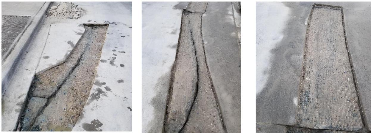
Figure 4 – Concrete pavement condition after milling and surface preparations
