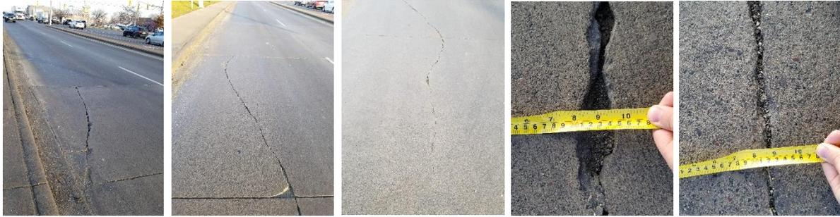
Figure 3 – Original condition of the concrete pavement
