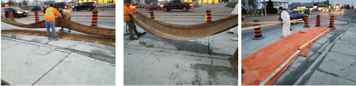
Figure 6 – Curing and protection procedure
