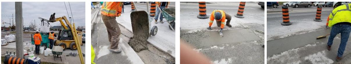
Figure 5 – Production and pouring of the patching repair materials
